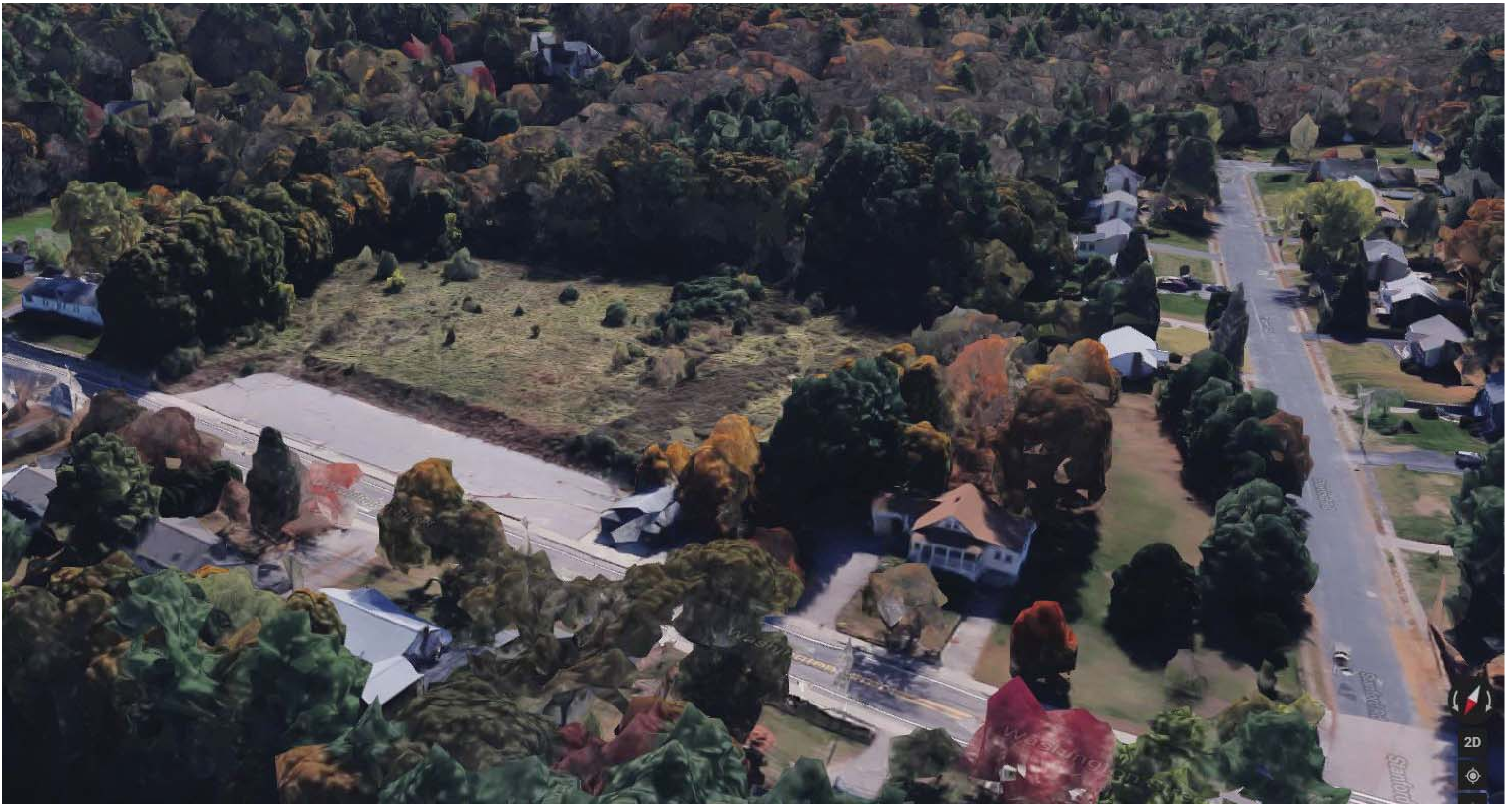
AERIAL VIEW OF EXISTING CONDITIONS
