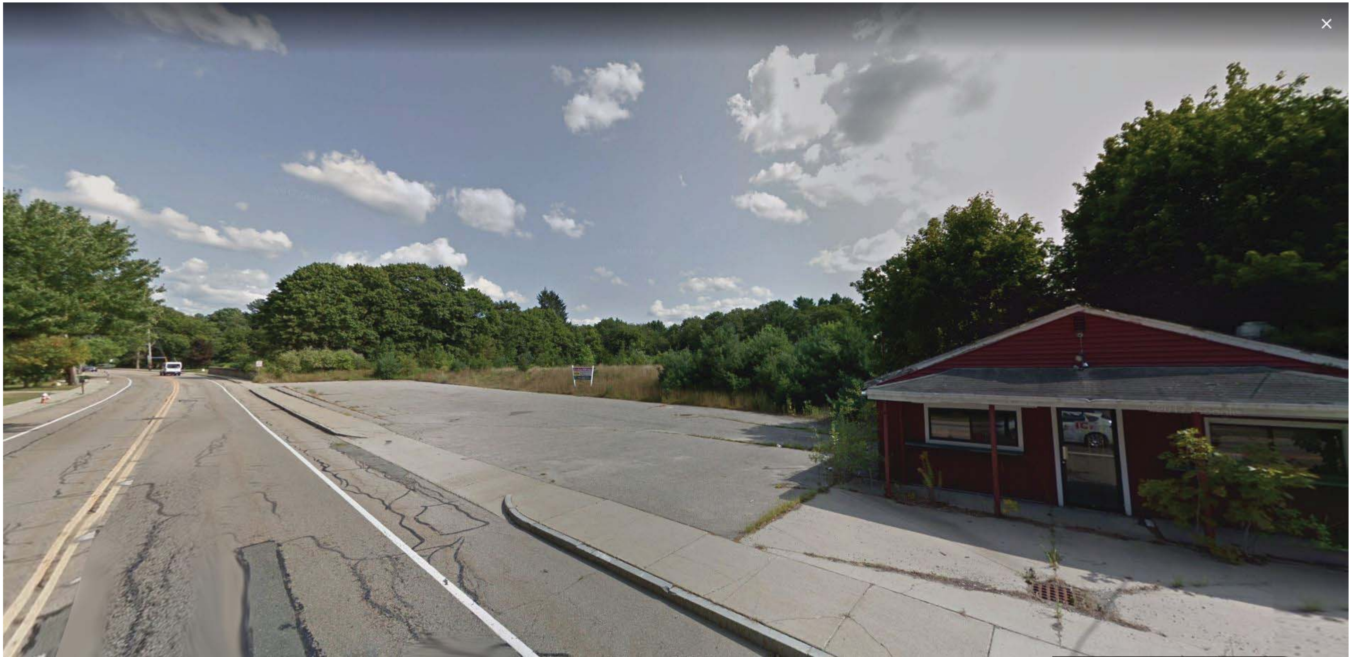
WASHINGTON STREET VIEW FACING SOUTHEAST- EXISTING CONDITIONS
