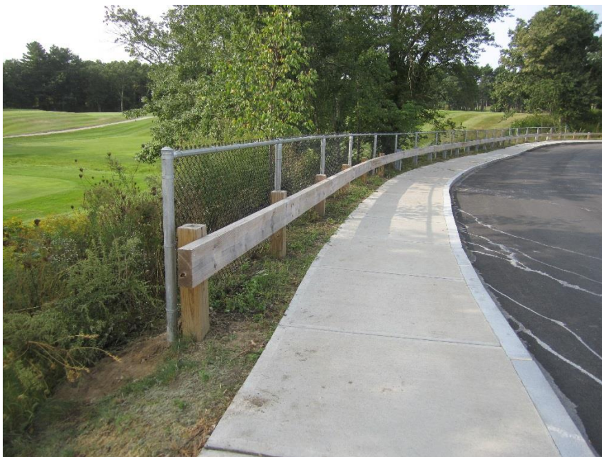
Safety fencing installed along Uncas Brook crossing retaining wall
