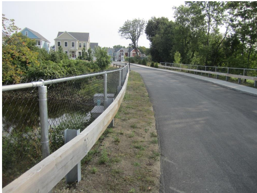
Safety fencing installed along Uncas Brook crossing retaining wall
