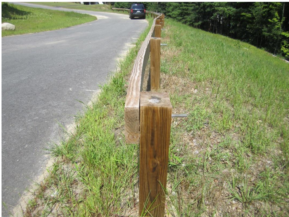
Installed guardrail
