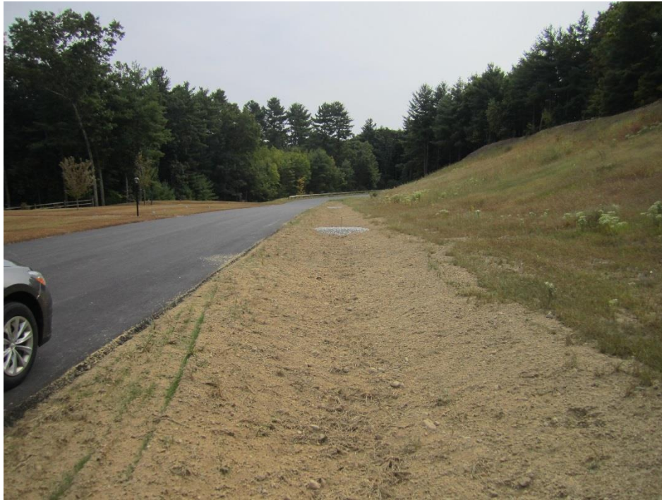
Recently seeded swale with check dams
