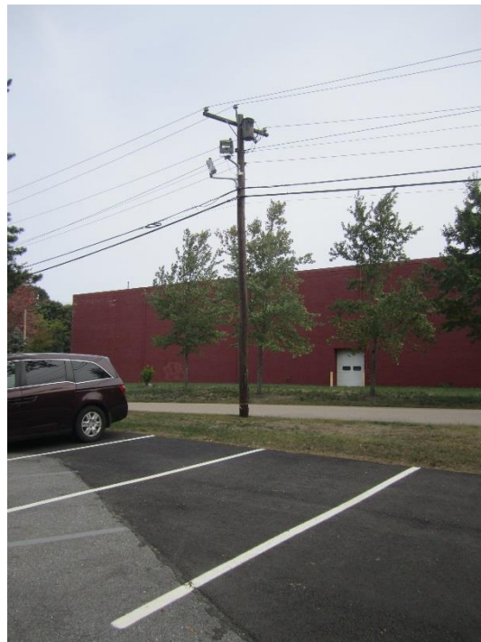
Flood light installation on Utility Pole 6
