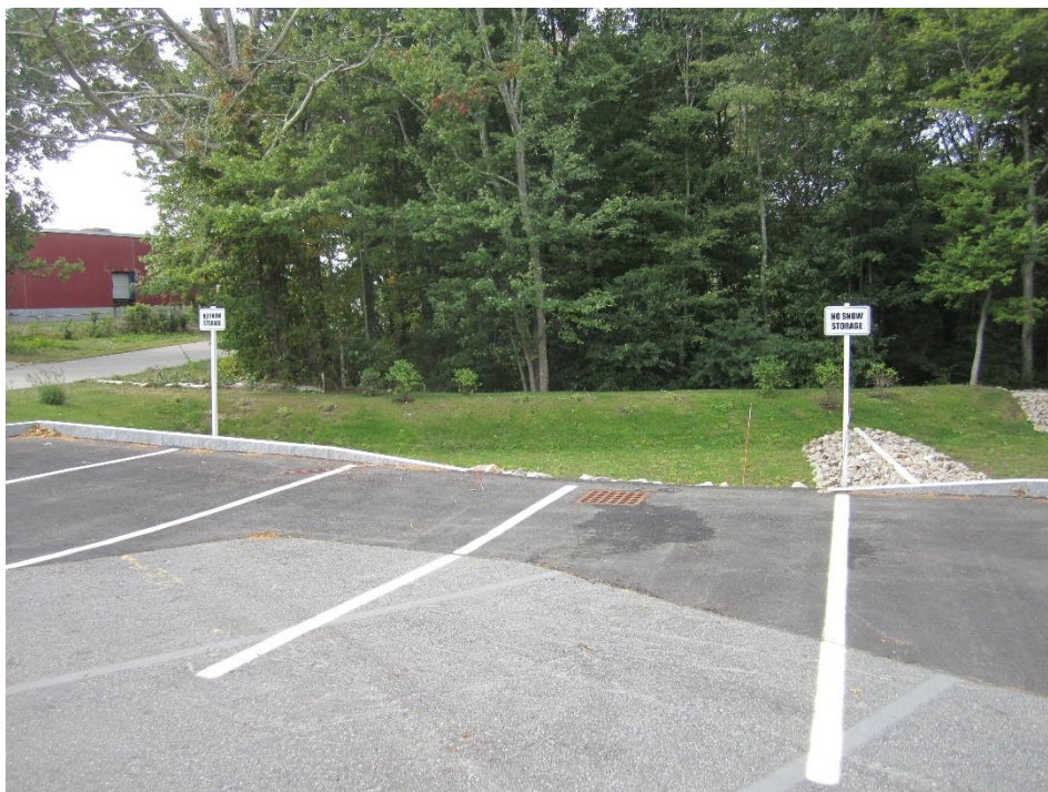
Area of consideration for guardrail or car stop installation
