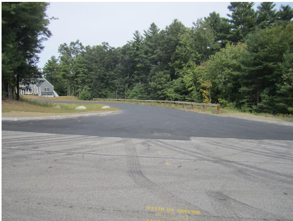
Constructed roadway at intersection of Brandywine Road
