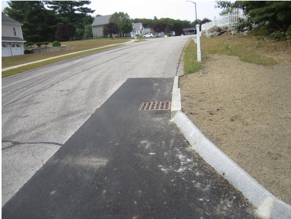
Installed radius stone and bituminous patch at Brandywine Road
