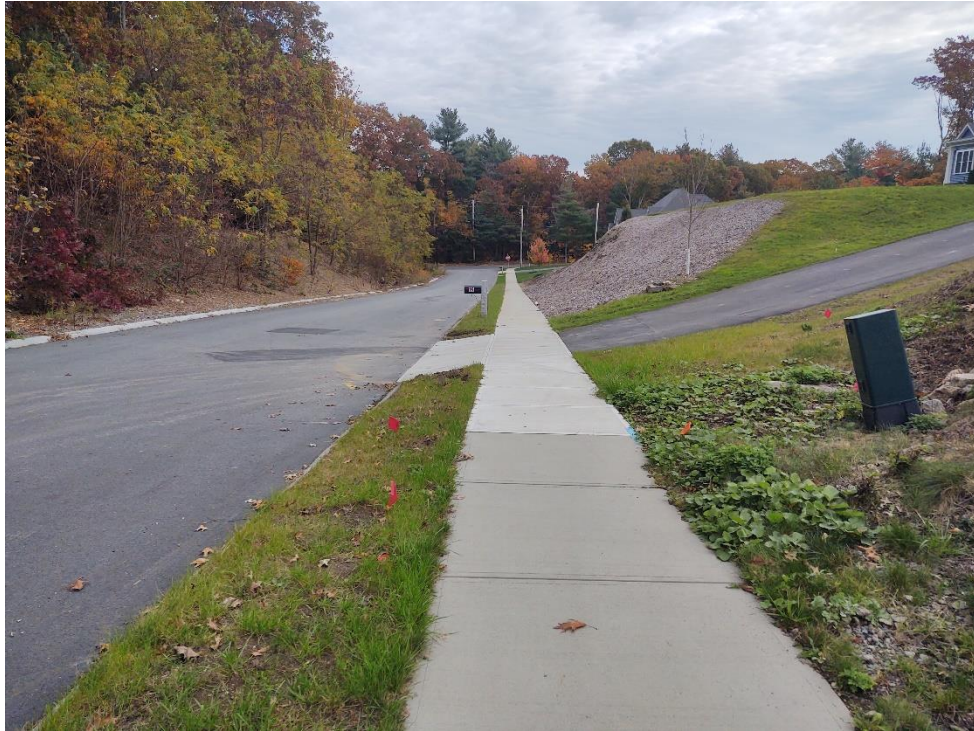
Recently completed work along Lot 1 frontage
