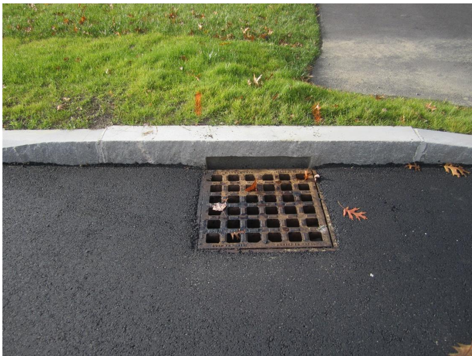
Typical drainage grate and inlet stone (photo 11/2021)
