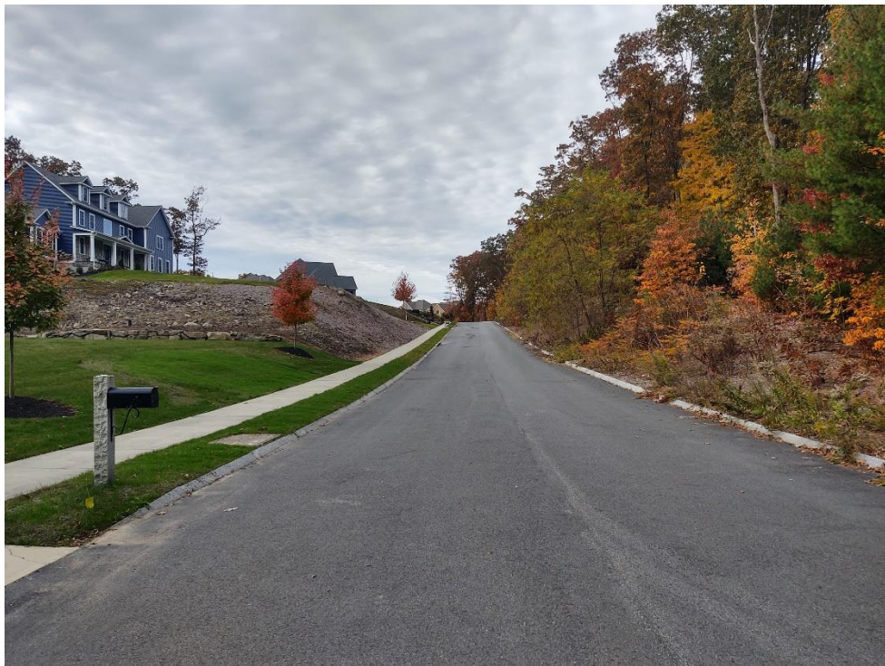
Typical Roadway, September Drive
