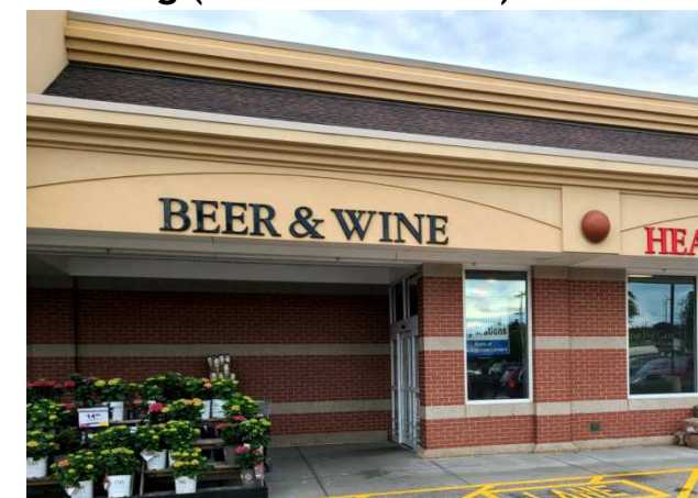
Existing ( to be removed )
