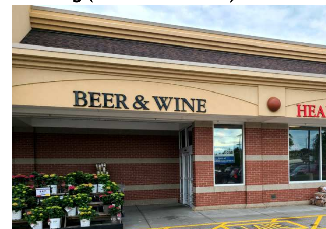
Existing ( to be removed )
