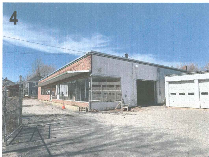
4 VIEW OF EXISTING BUILDING FACADE
