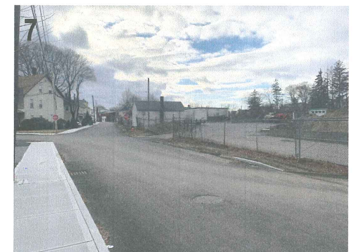
7 VIEW TOWARD INTERSECTION OF ALPINE ROW & ALPINE PLACE
