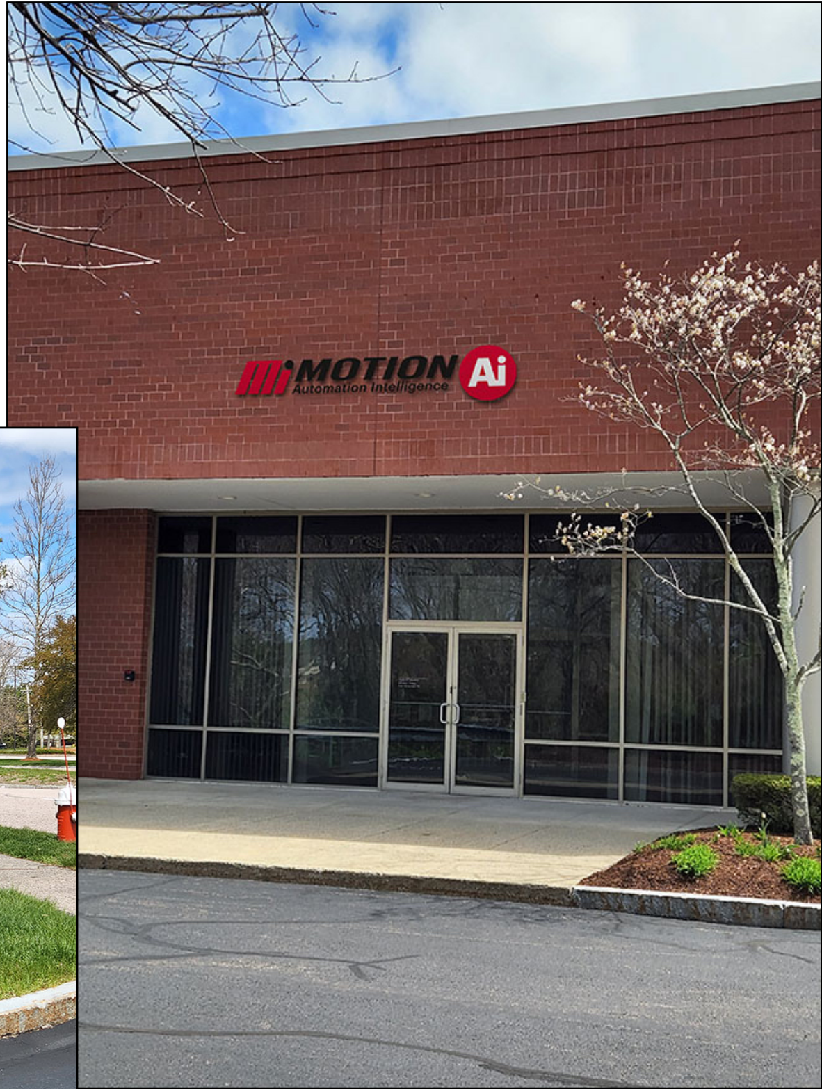
FRONT OF BUILDING
