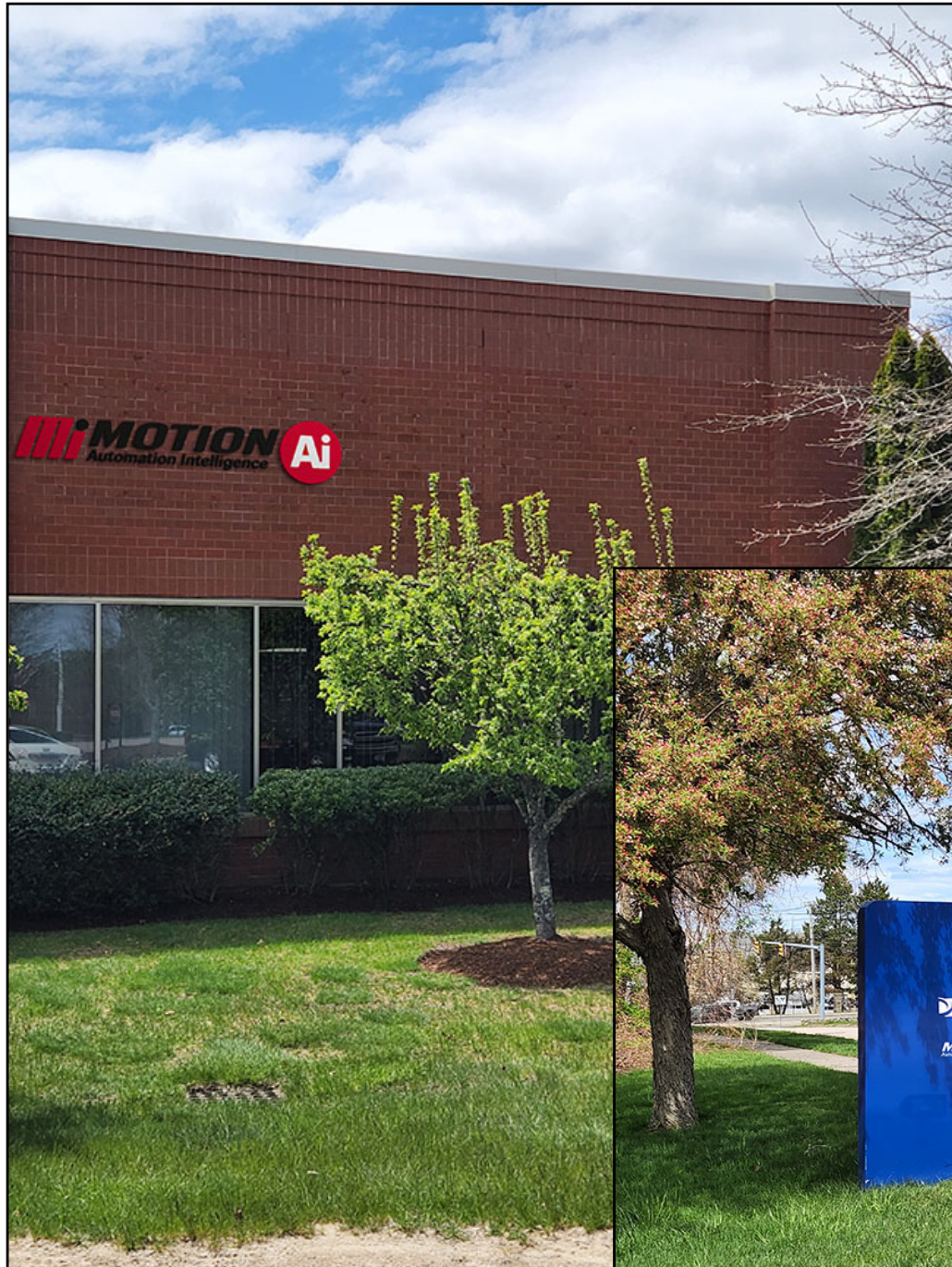
SIDE OF BUILDING
