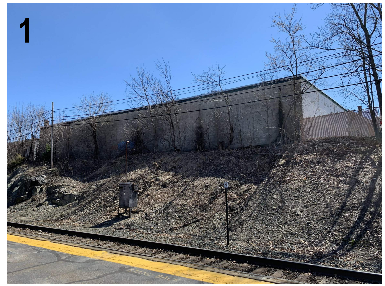
1 VIEW FROM COMMUTER RAIL PLATFORM
