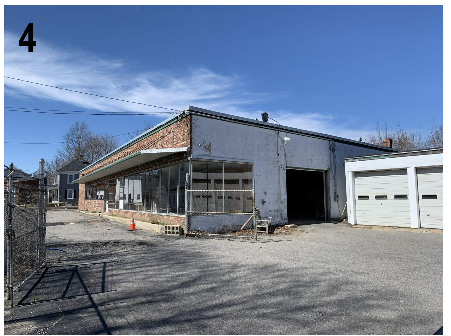
4 VIEW OF EXISTING BUILDING FACADE
