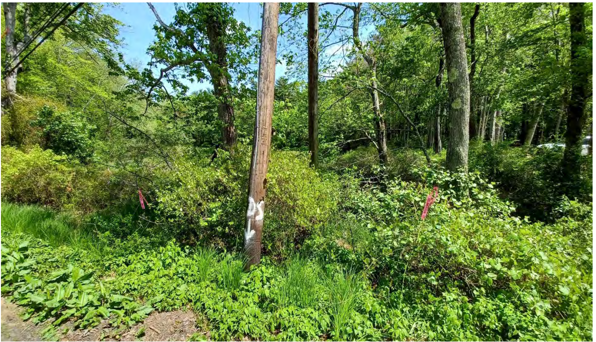
Photo #1: View of existing P49 and push-brace within BVW. The pole is proposed to be replaced in-kind, and the push-brace permanently removed. Facing northeast.
