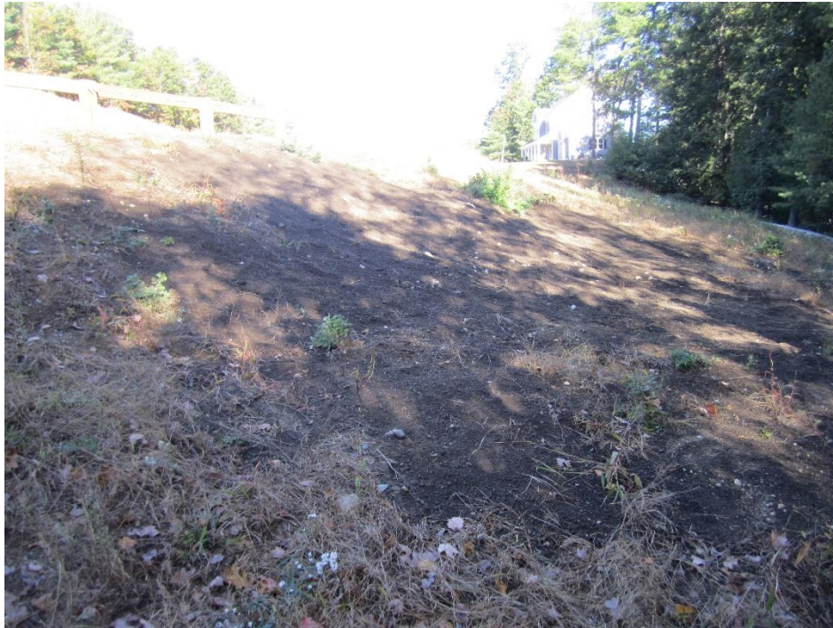
Repair of eroded slope
