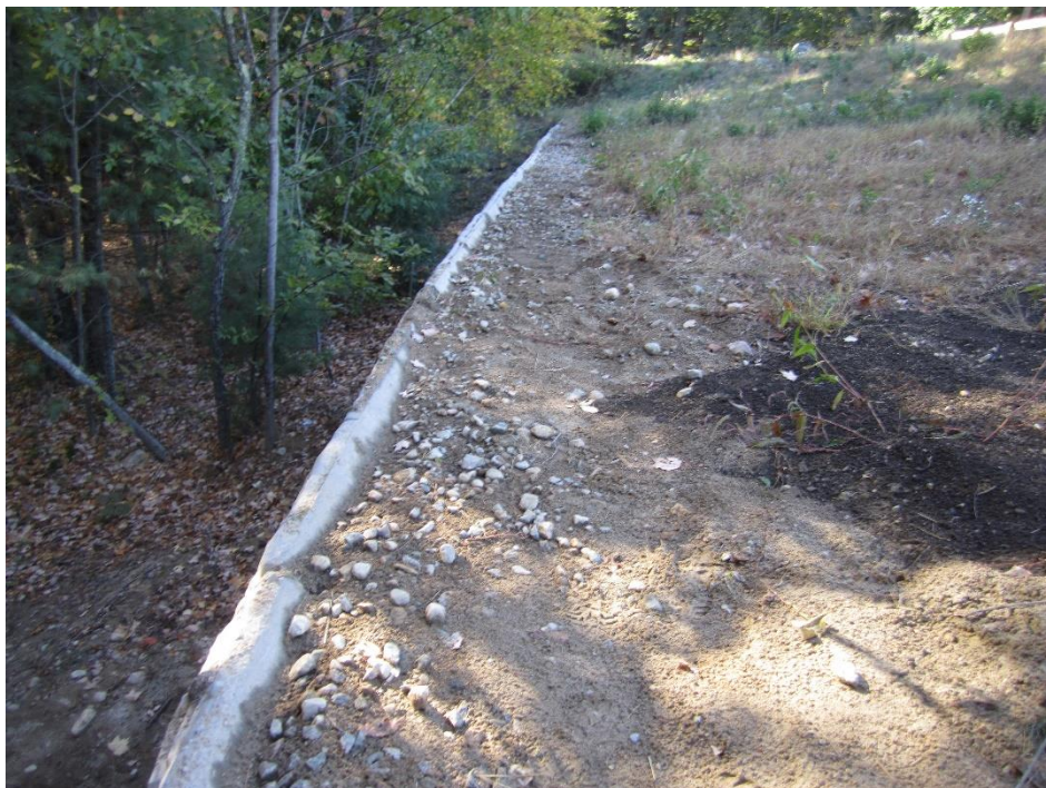
Revised grading at top of retaining wall
