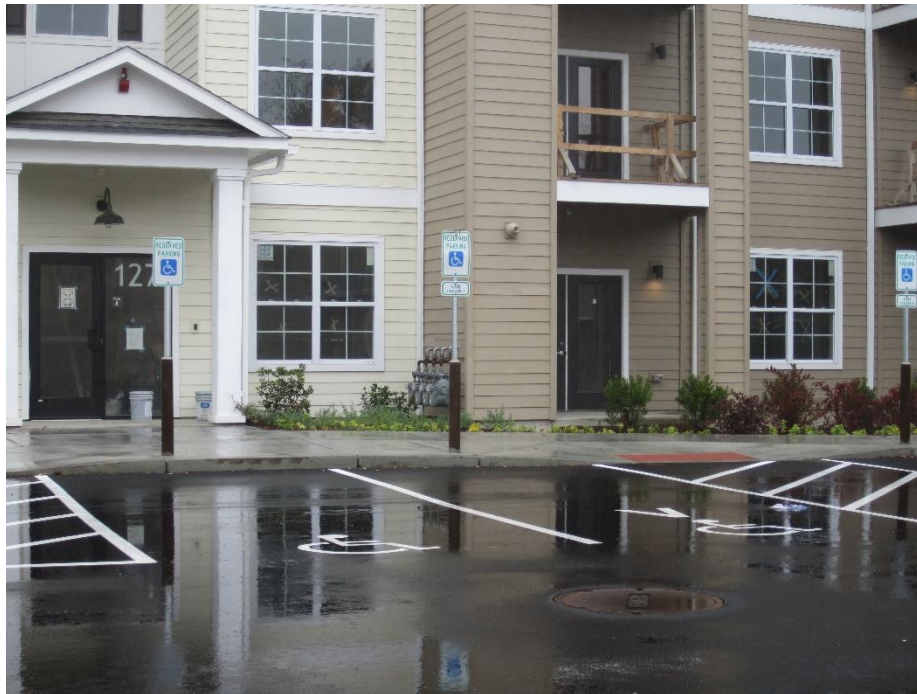
Typical accessible parking at building entrance
