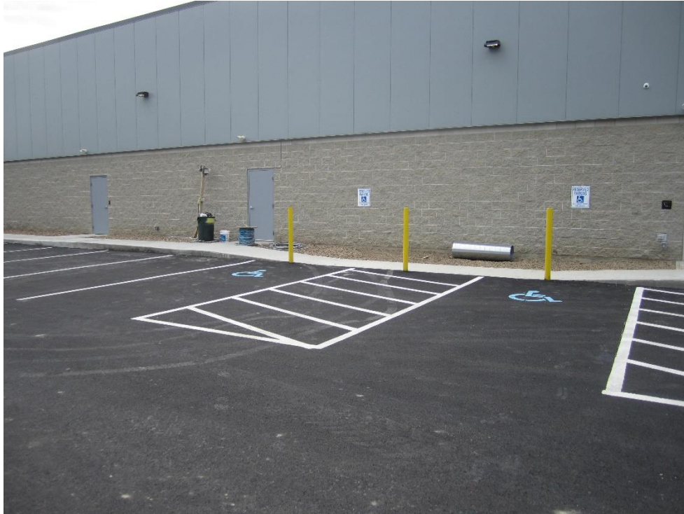
Bollards installed at flush sidewalk
