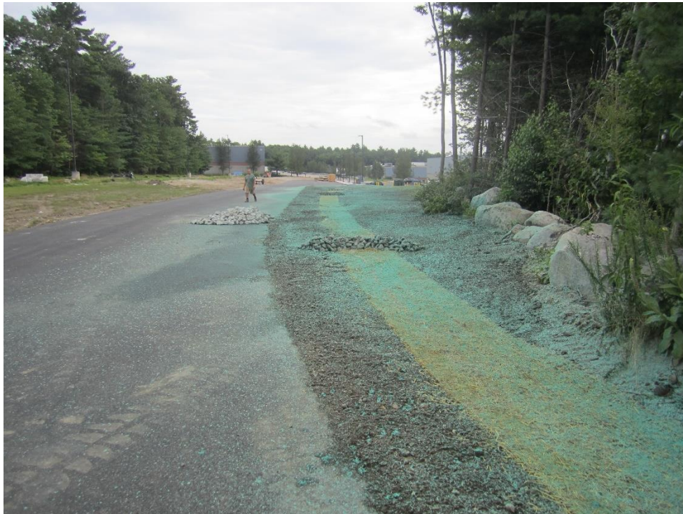
Drainage swale and rip rap installation
