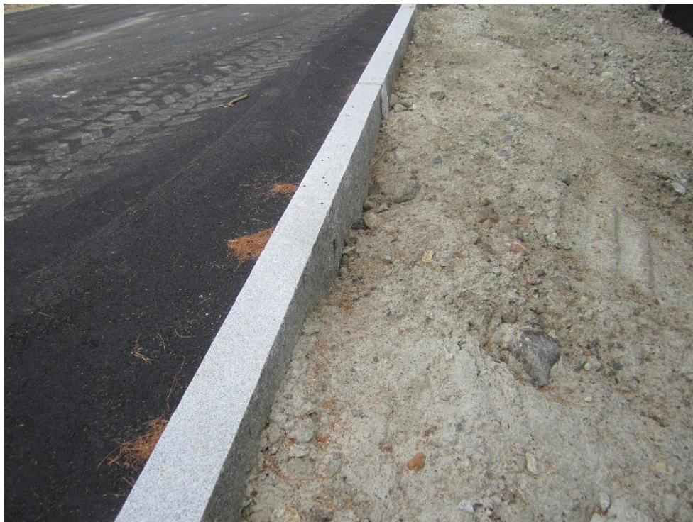
Typical area behind curb requiring fill, loam, and seed
