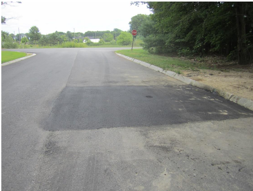
Utility patch on Liberty Way that has been bonded with infrared
