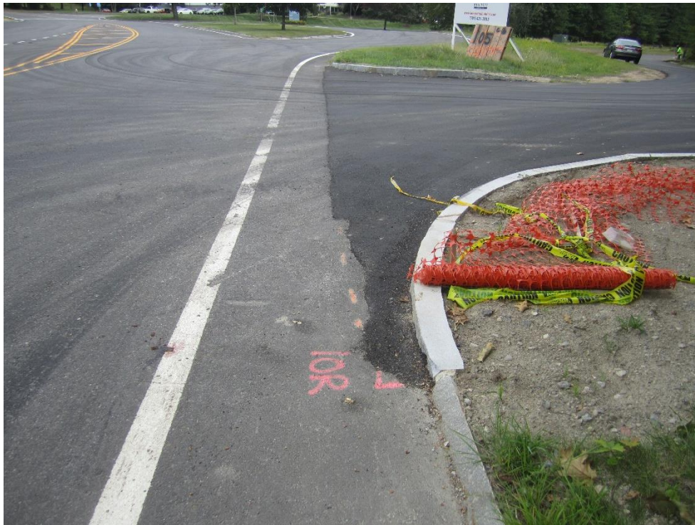
Granite curb radius at site entrance
