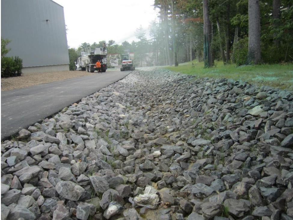
Drainage swale adjacent to roadway
