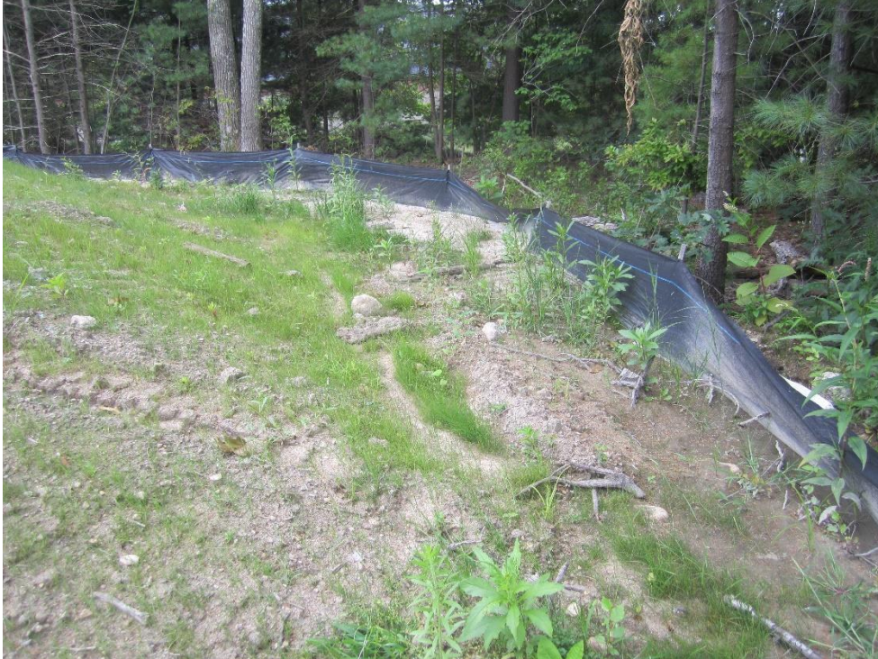
Typical silt fence that requires removal after full site stabilization
