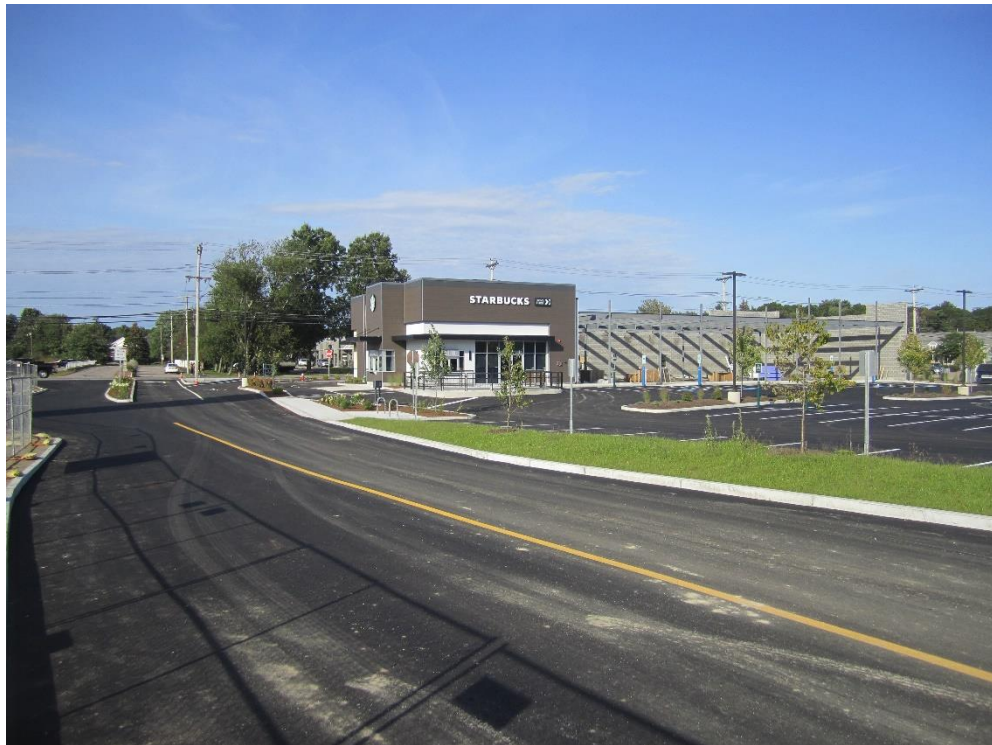
Site driveway and Building C
