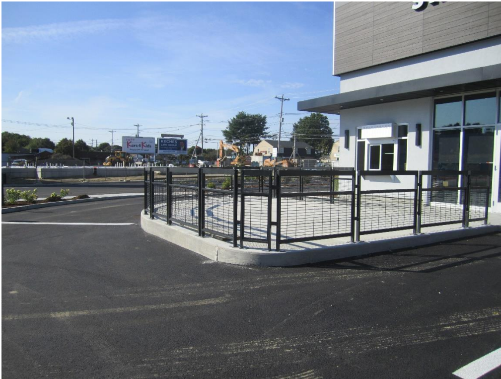
Concrete patio and fence installed at Building C
