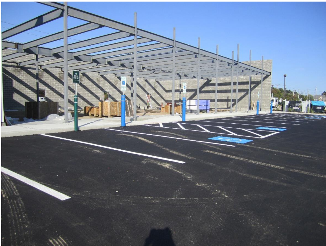
Accessible parking at front of Building C
