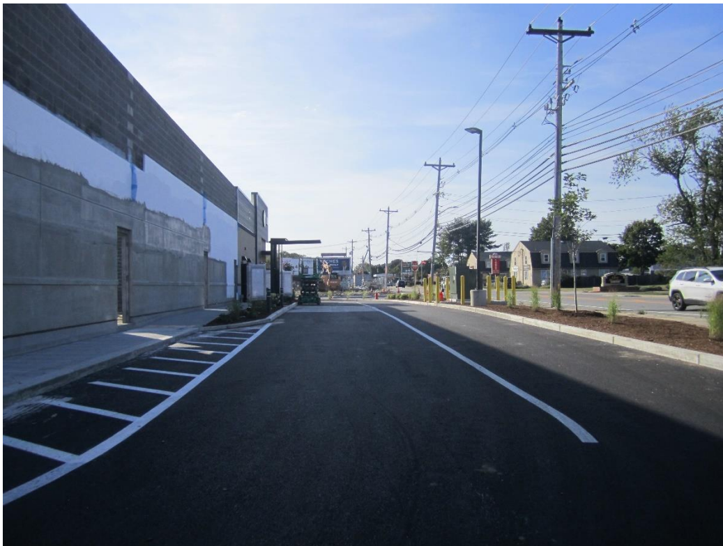
Damaged light pole to be replaced
