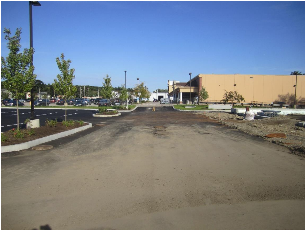
Site driveway paved to binder course with raised castings
