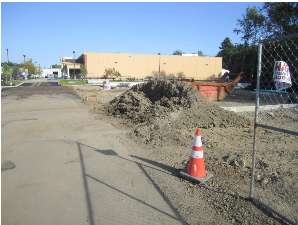
Limits of construction fencing at time of visit.
