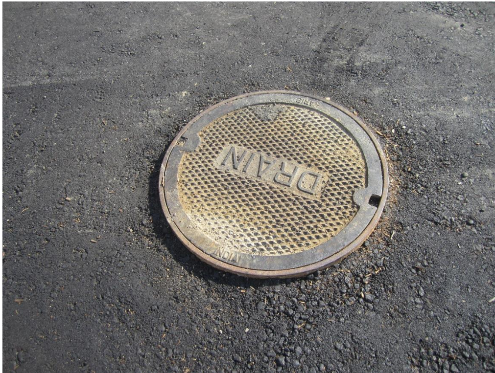
Foreign made casting that requires replacement with domestic casting
