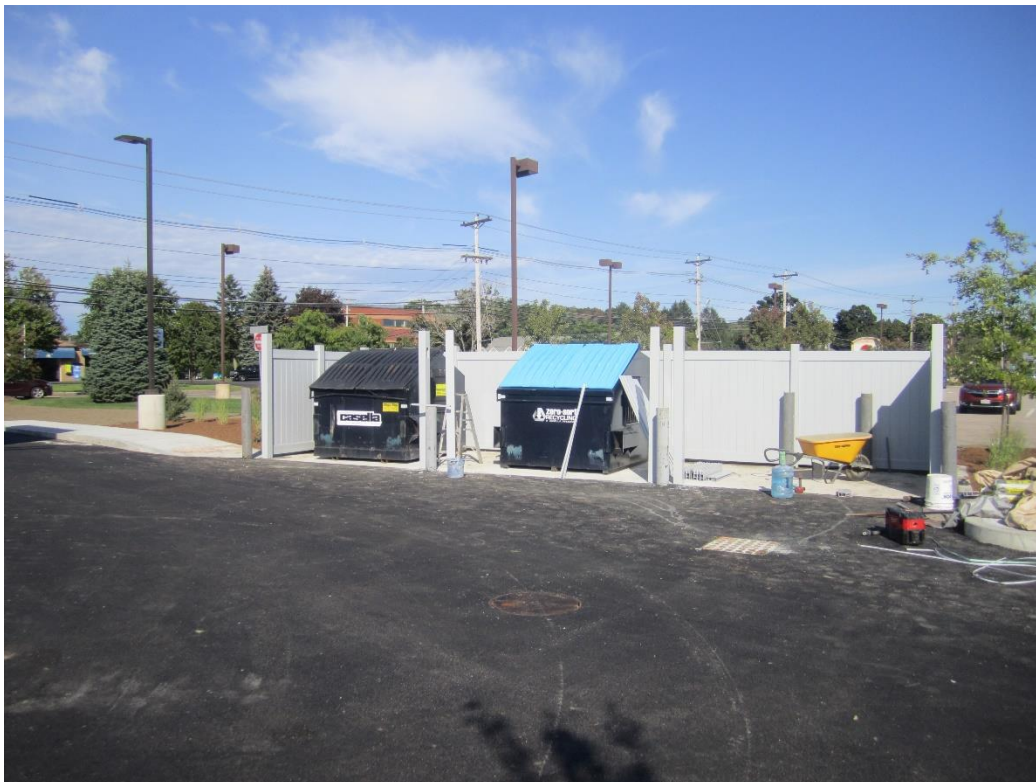
Dumpster enclosure currently under construction
