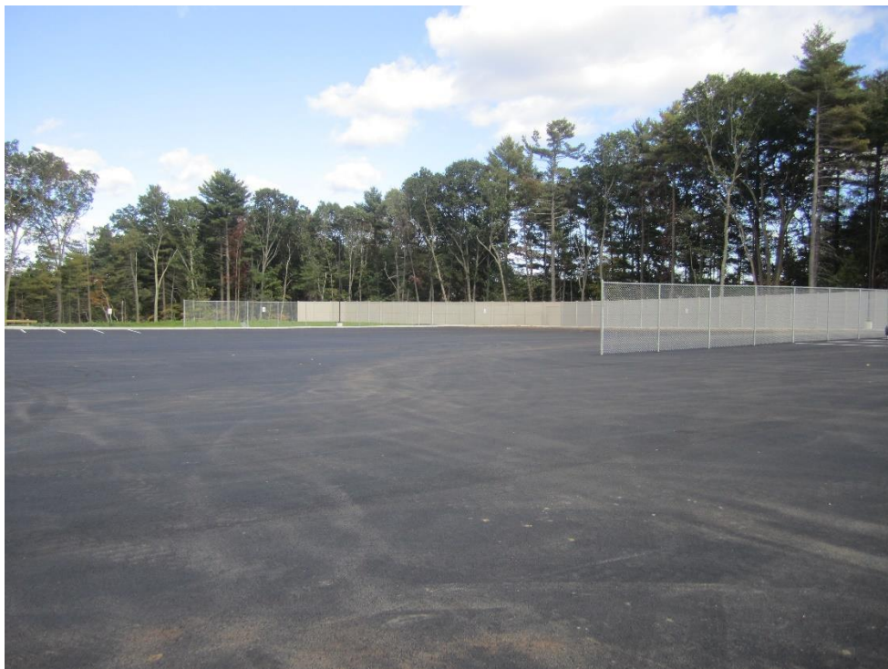
New/reconstructed pavement area
