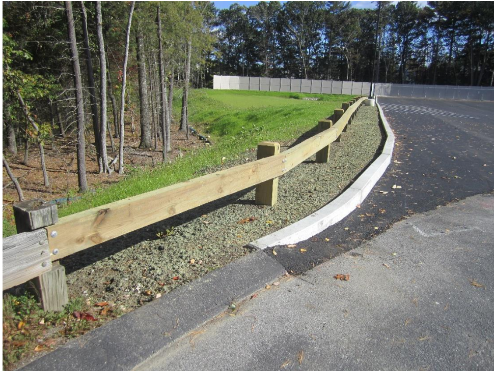
Typical curb and wooden guardrail installation
