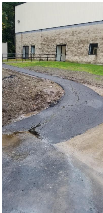
Reconstructed walkway ( photo provided by contractor )
