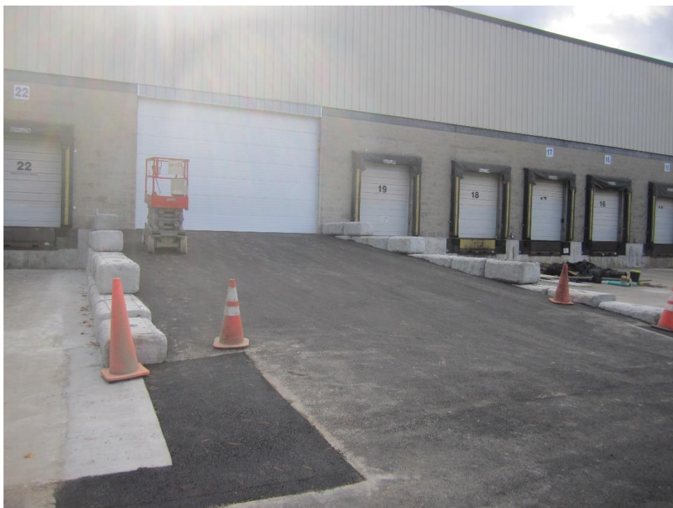
Ramp access to building
