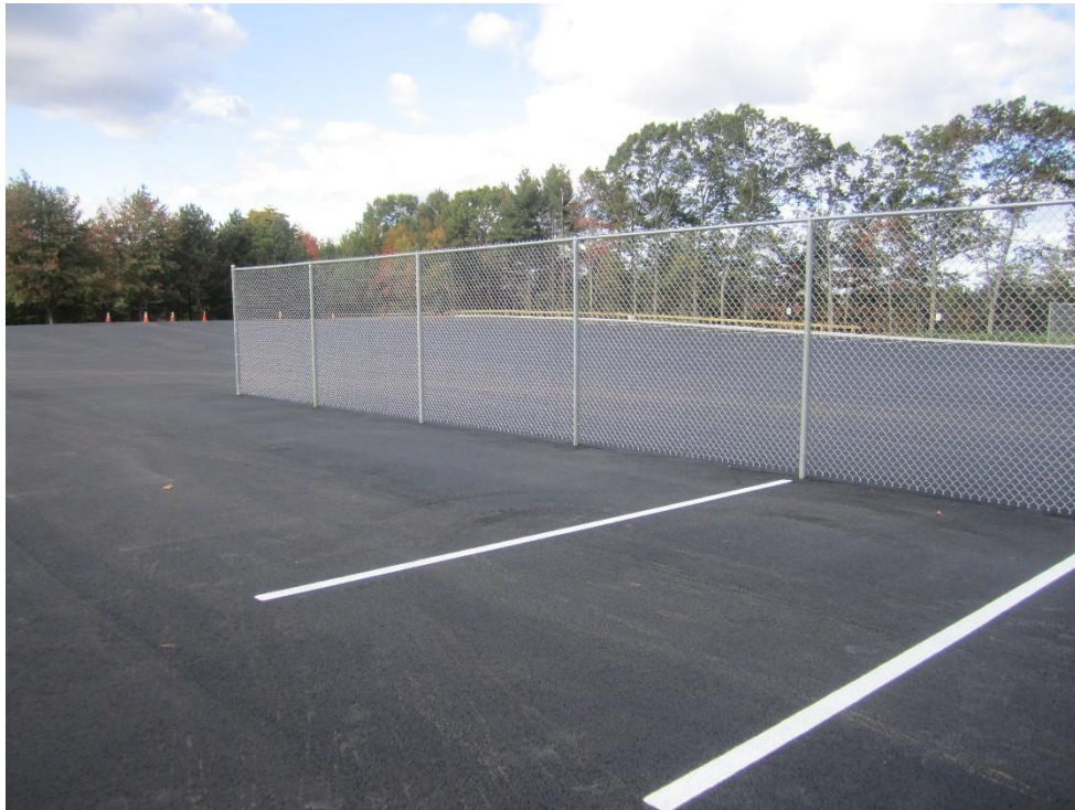
Fencing separating parking and storage areas
