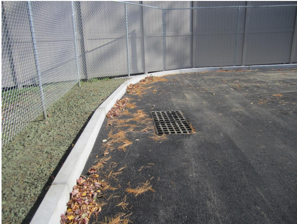
Installed drainage structure, located at low point
