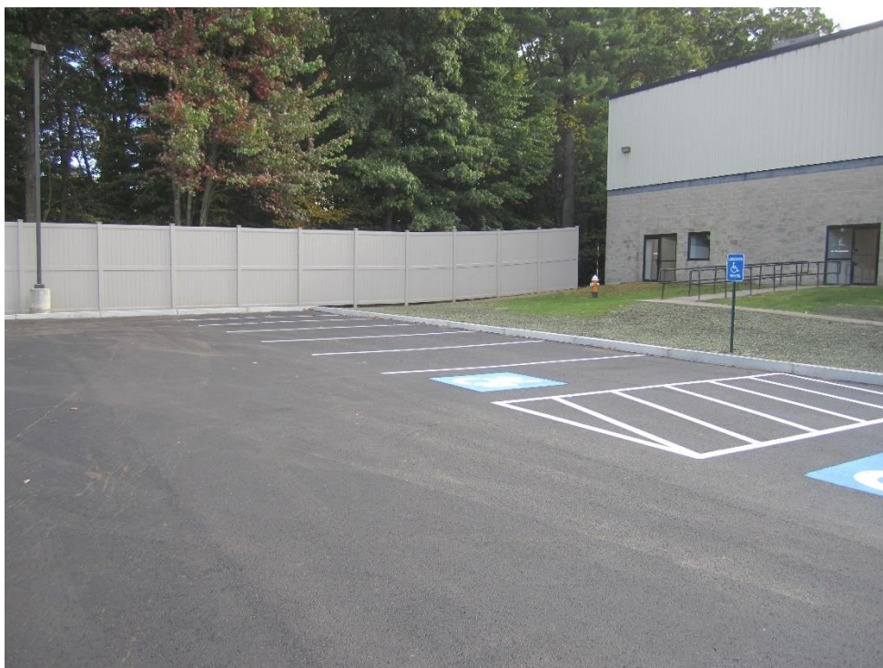
Screening fence extending to building
