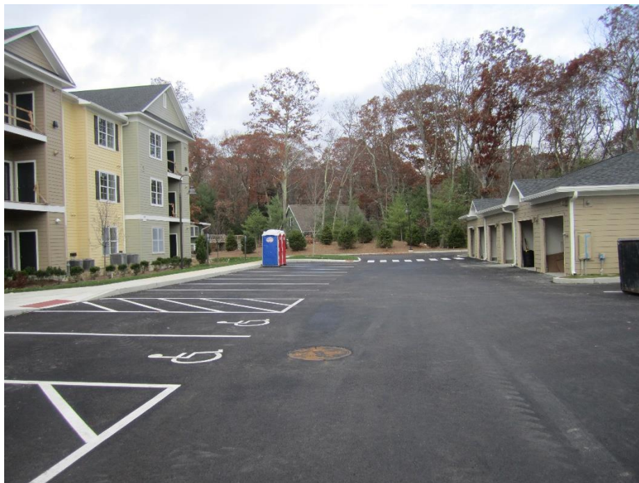
Parking area between Building 6 and Garage 9
