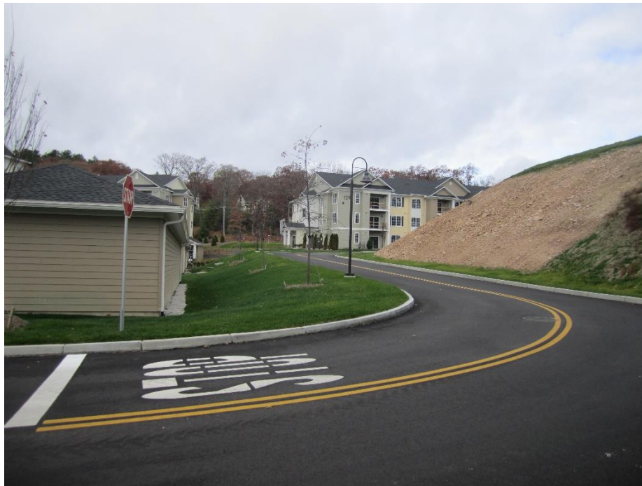
Guardrail has not been installed along the roadway between Buildings 5 and 6
