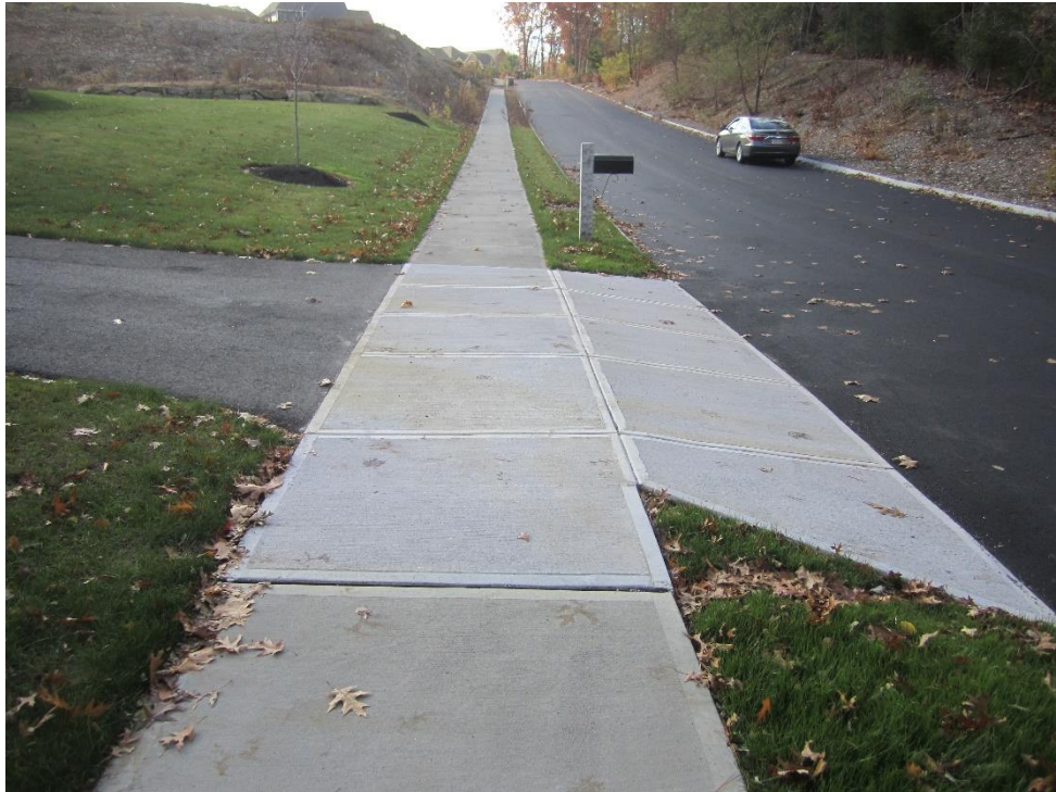
Typical sidewalk and concrete apron installation
