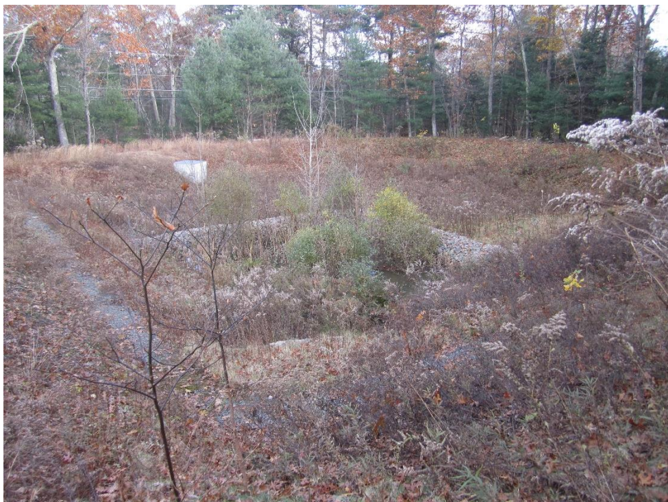
Woody vegetation in Infiltration Basin No. 1 that requires removal
