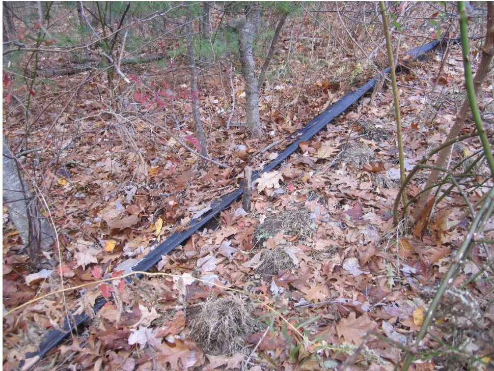
Typical silt fence that requires removal
