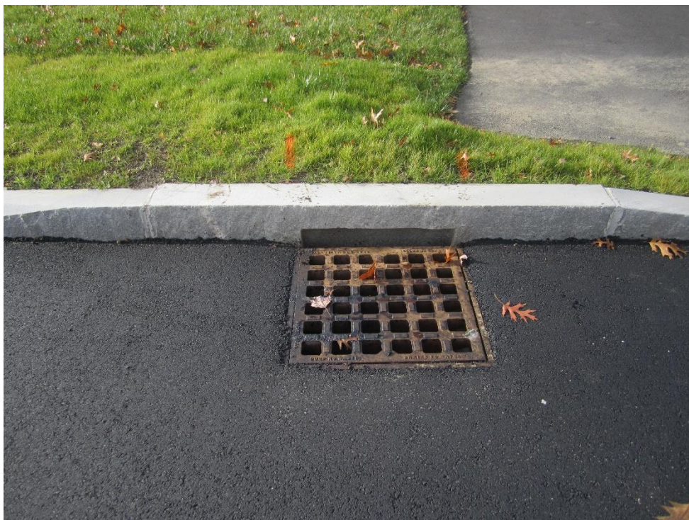
Typical drainage grate and inlet stone
