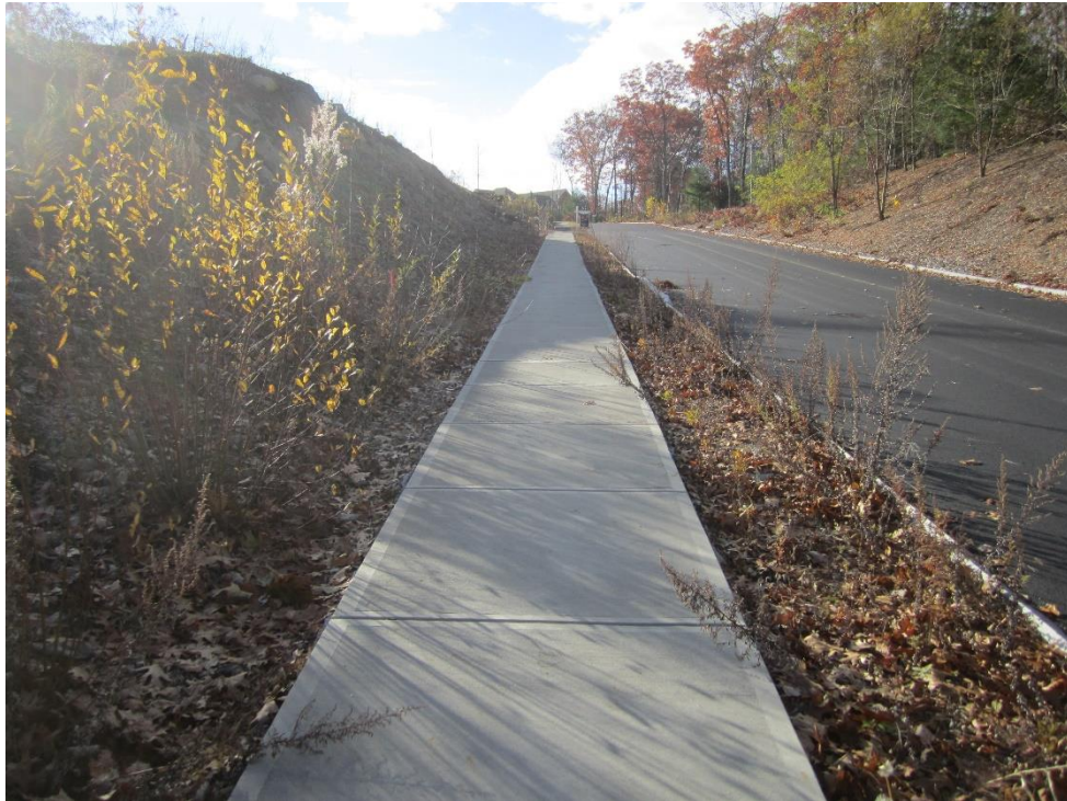
Area along Lot 1 frontage that requires loam and seed installation
