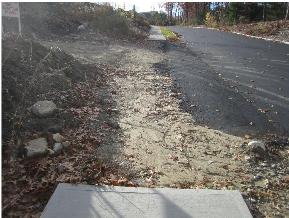
Area along Lot 1 frontage that requires sidewalk, curb, and driveway installation
