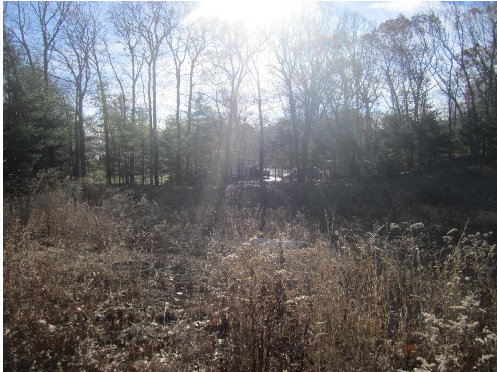
South side of Infiltration Basin No. 1 lacking screening
