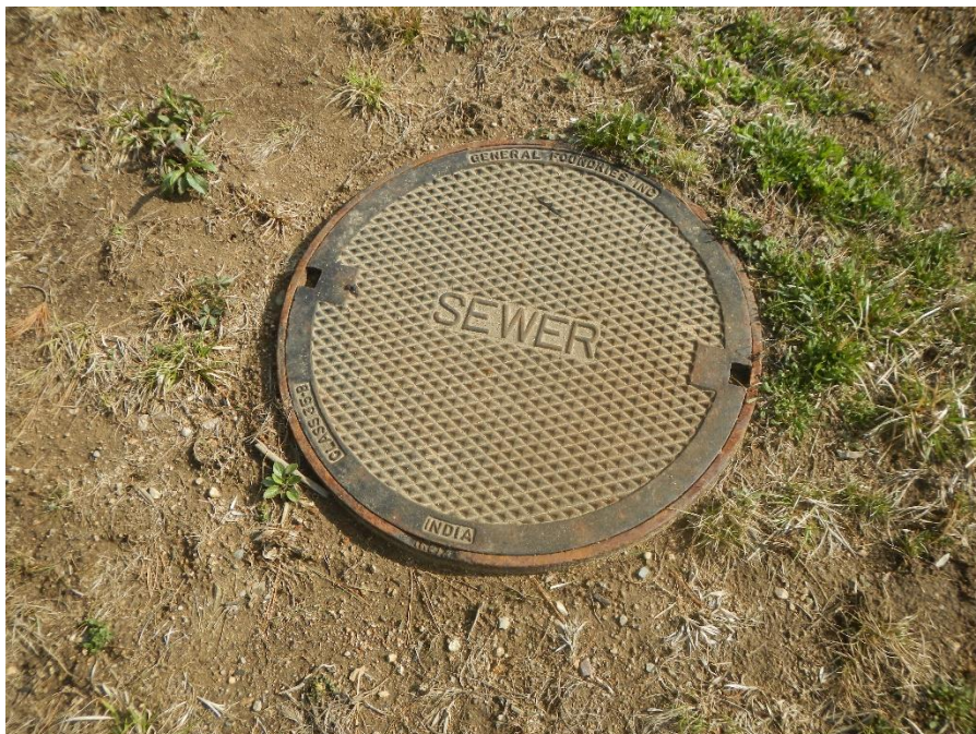
"India" casting near pump chamber
