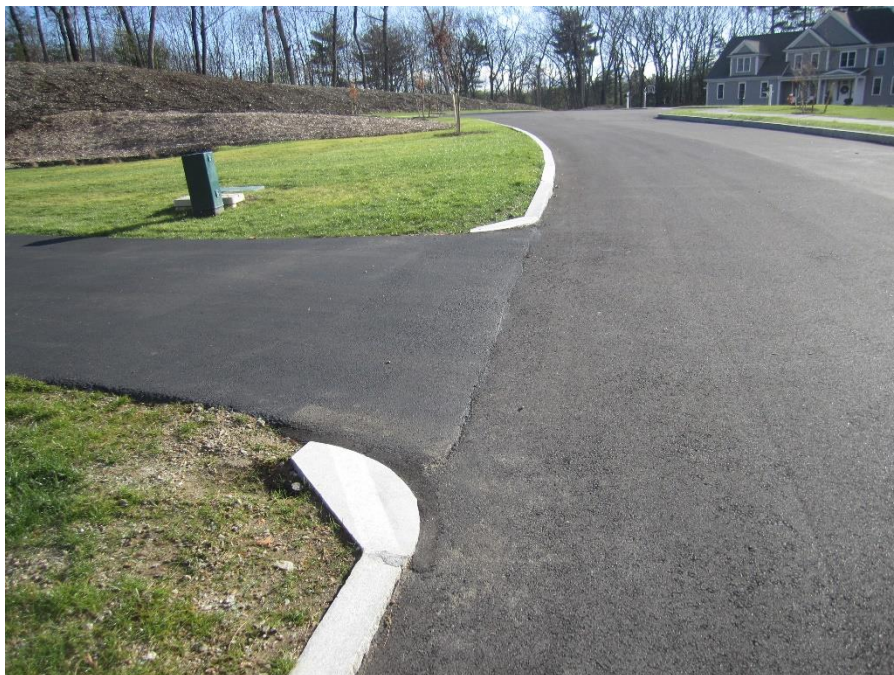
Installed granite radius stones with minimal reveal
