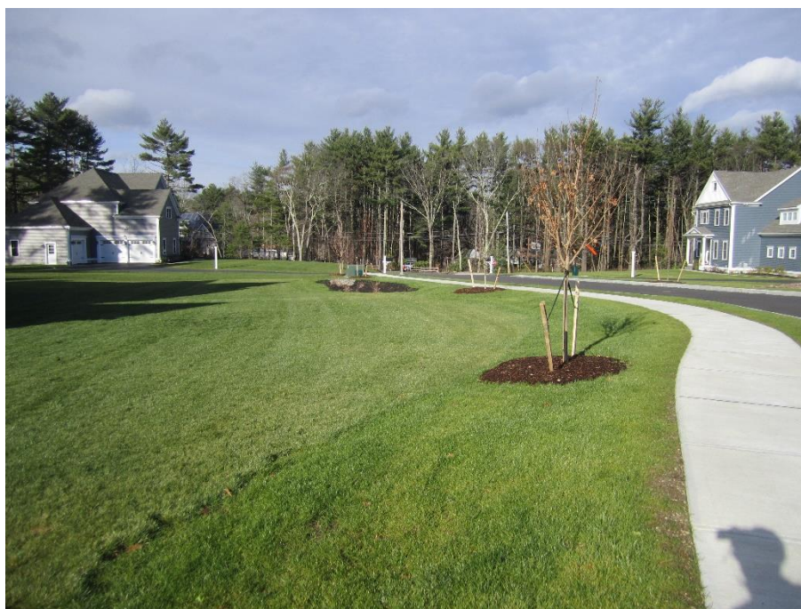
Grading revised between sidewalk and residential lots to make a mild transition
