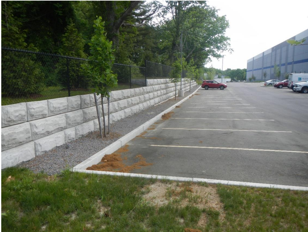
Northerly parking and retaining wall
