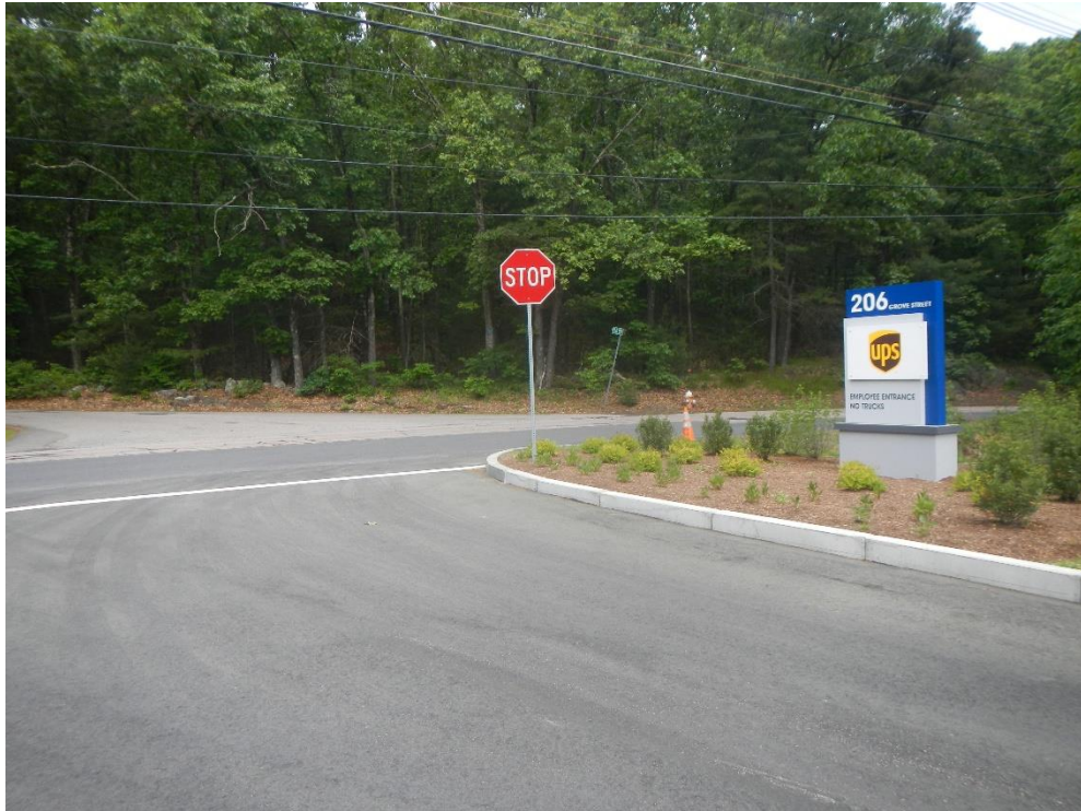
Site entrance and signing
