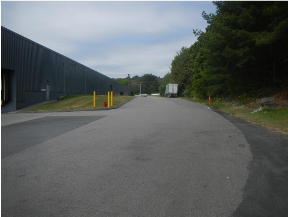
Unmodified access drive along #210 Building
