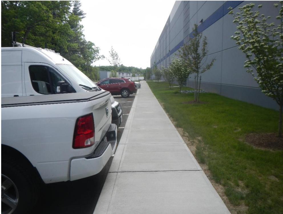
Typical sidewalk installation
