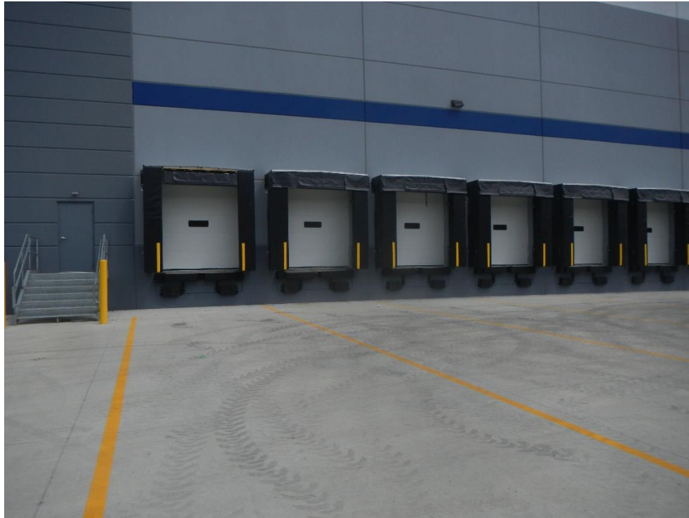
Typical loading dock installation
