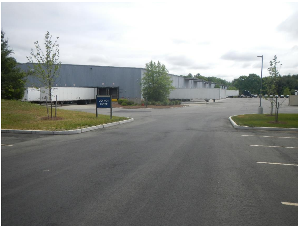
Driveway lacking security gates, replaced with "Do Not Enter" signage.
