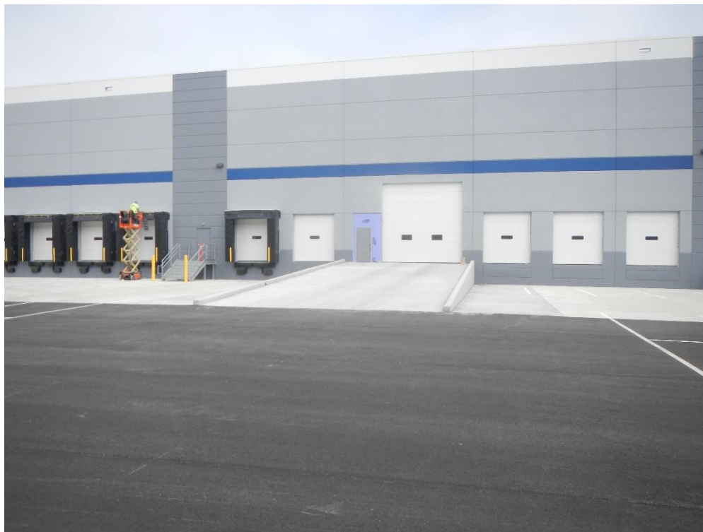
Additional drive-in ramp added
