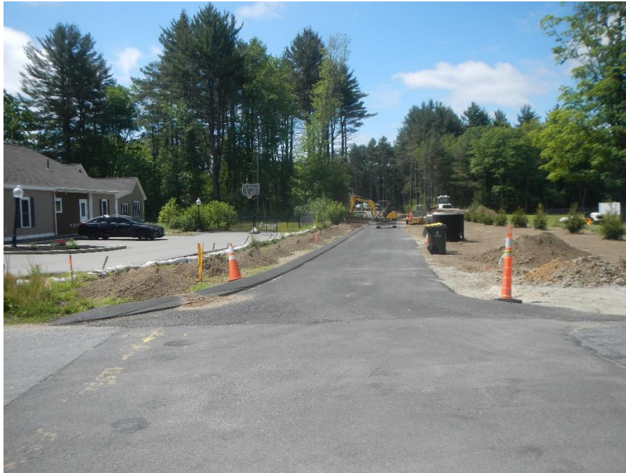
Subdivision roadway, showing binder course and Cape Cod Berm
