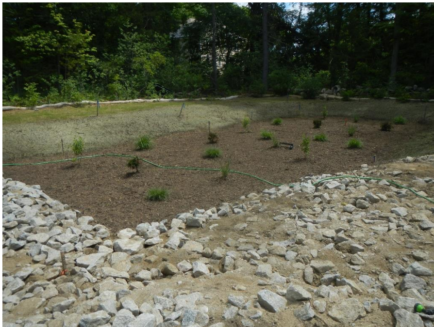
Completed rain garden area
