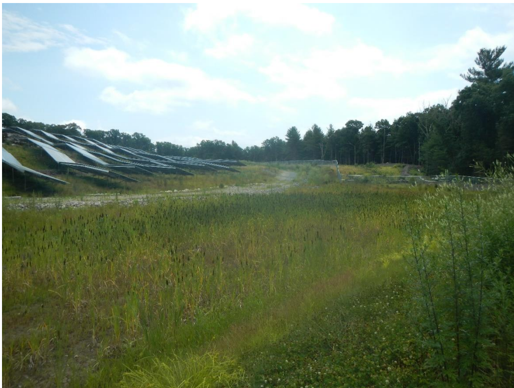
Infiltration Basin No.1, which requires maintenance and restoration
