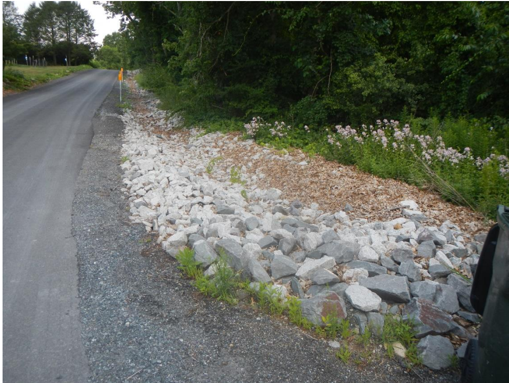
Sediment basin at base of Spring Street Paving
