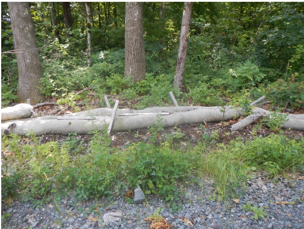
Typical perimeter erosion controls that remain in place
