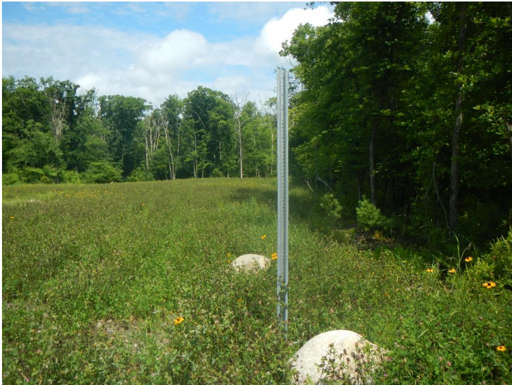
Sign post missing accessible signage. Restored laydown area shown in background.
