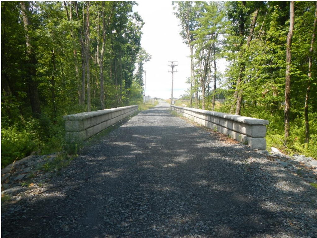
Access road at wetland crossing with retaining walls
