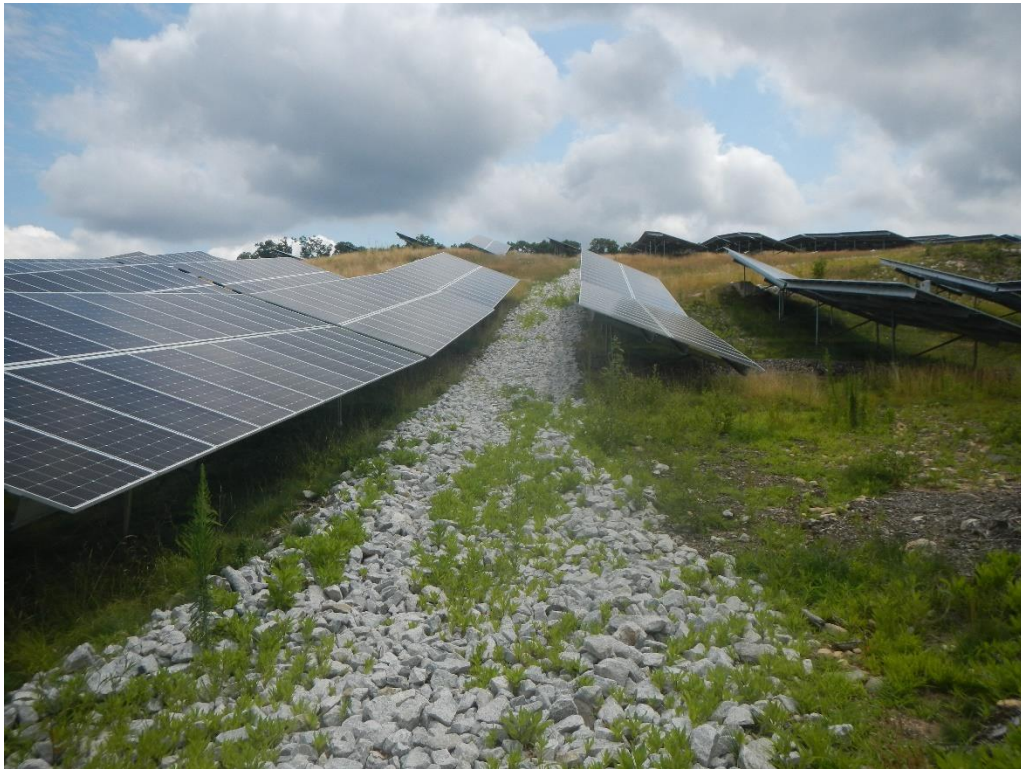
Rip rap swale installed for site stabilization
