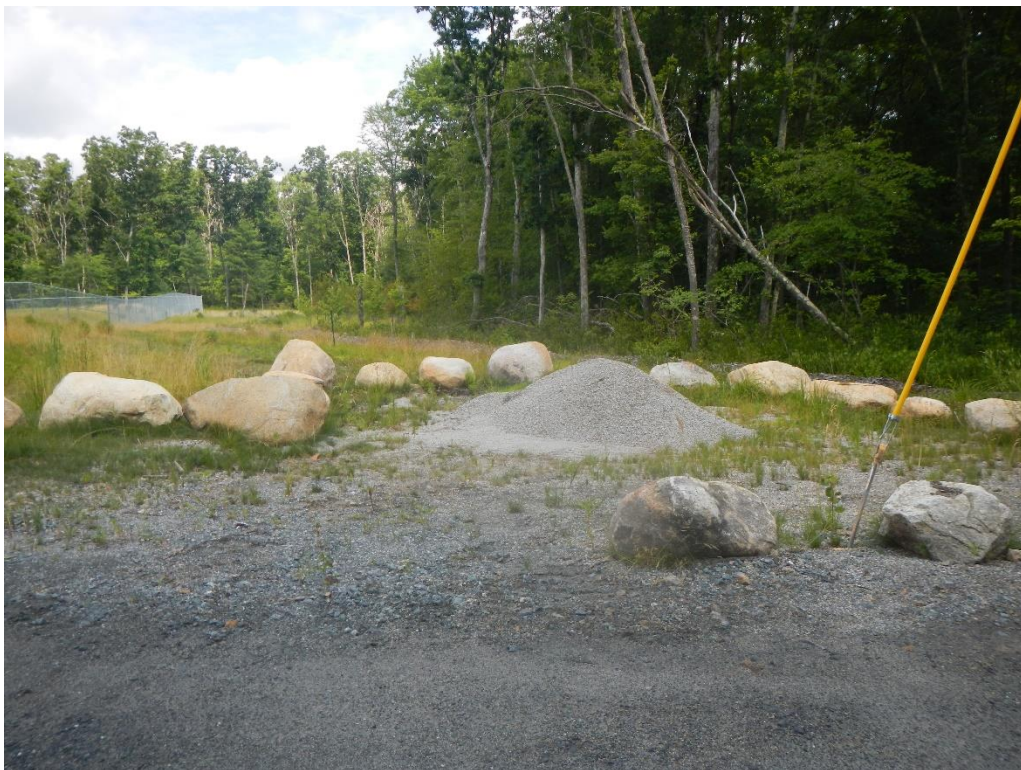
Hammerhead near main access gate, partially blocked, and with gravel stockpile
