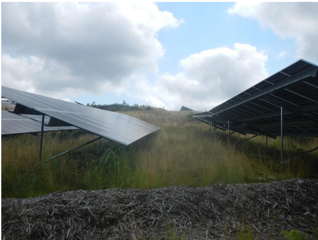
Typical stump grinding berm
