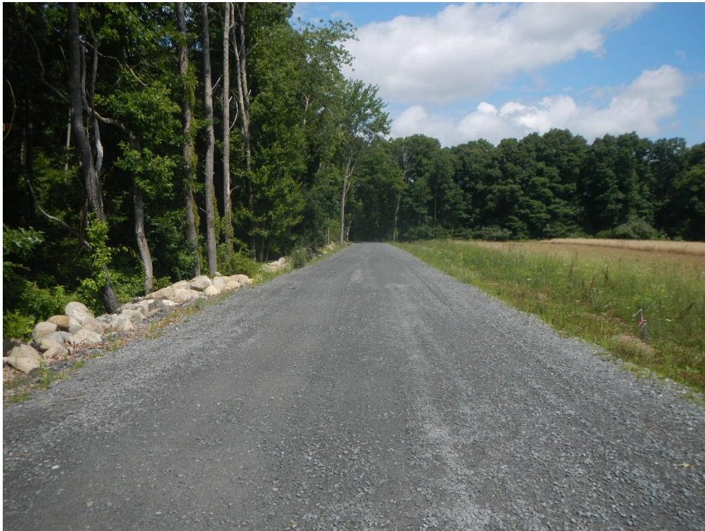
Typical processed gravel section of Spring Street
