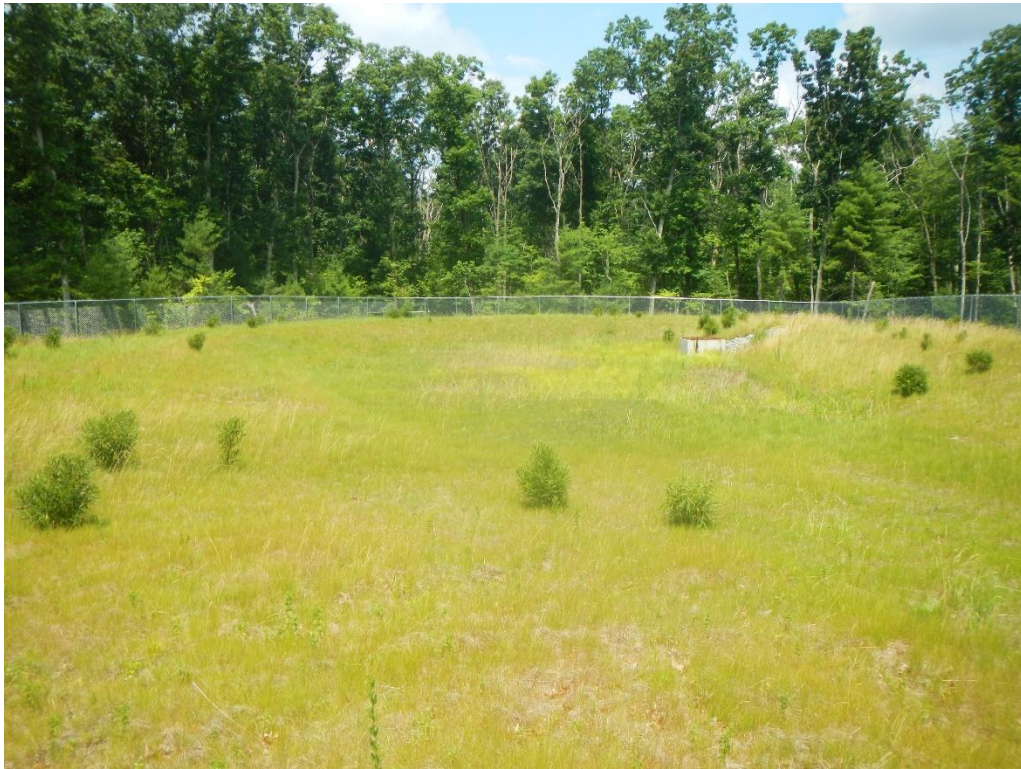
Infiltration Basin 2 – vegetated and operating as designed
