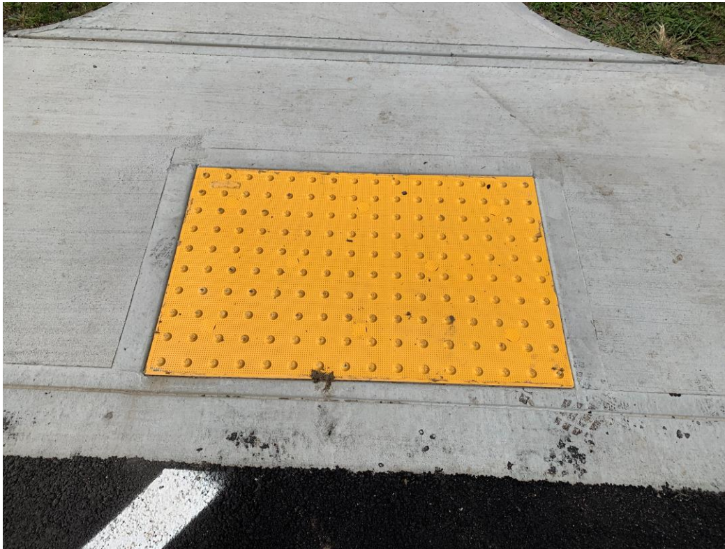
Detectable Warning Panel (Typ.)
