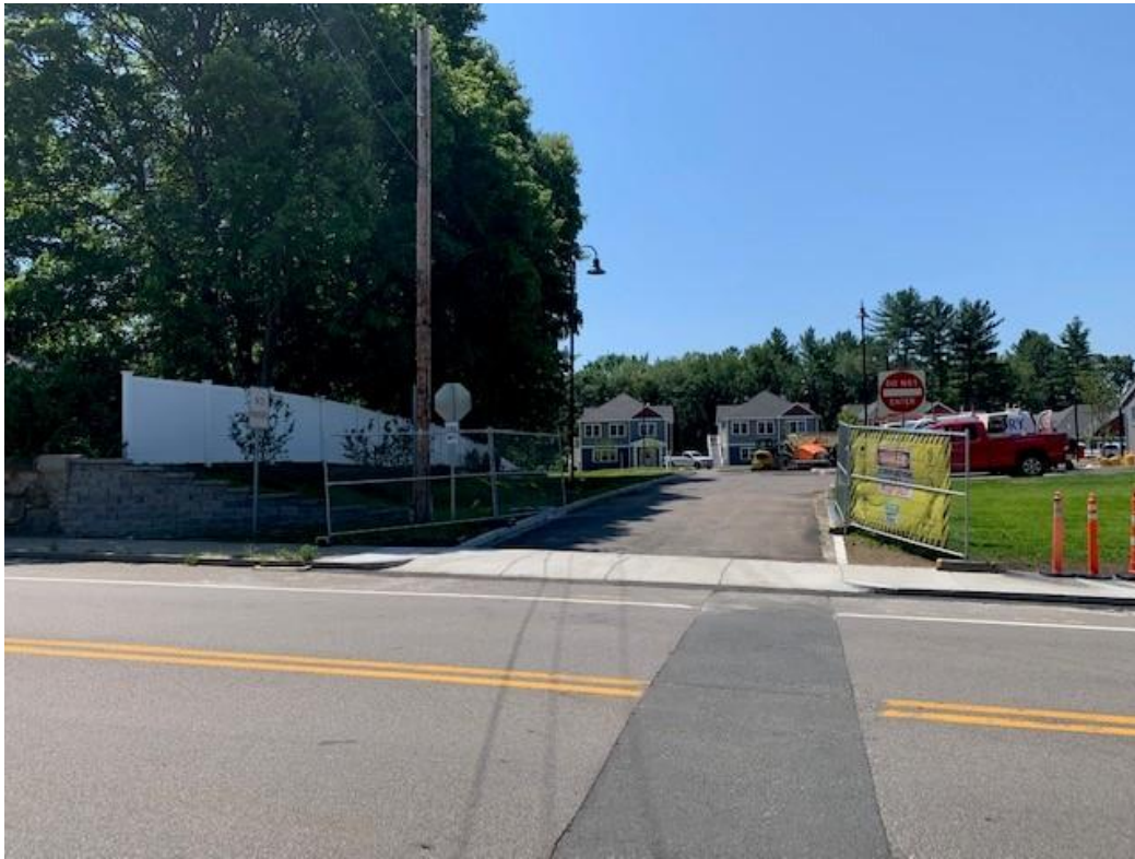
Easterly site entrance and signage
