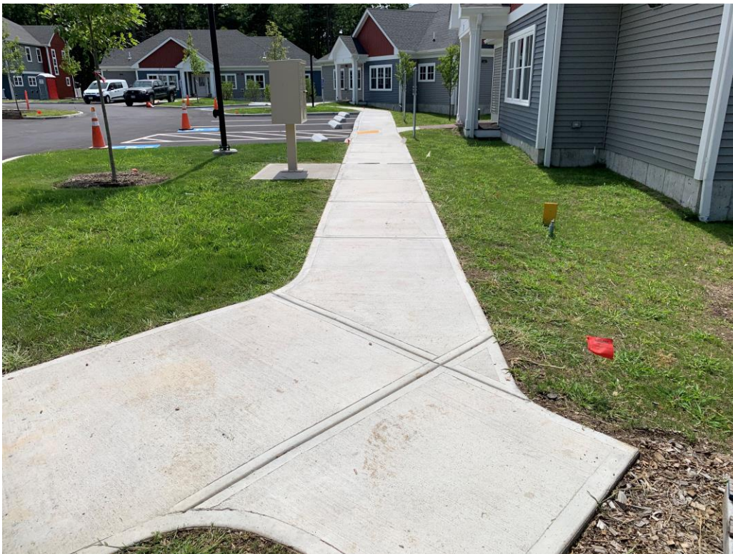
Typical Concrete Sidewalk
