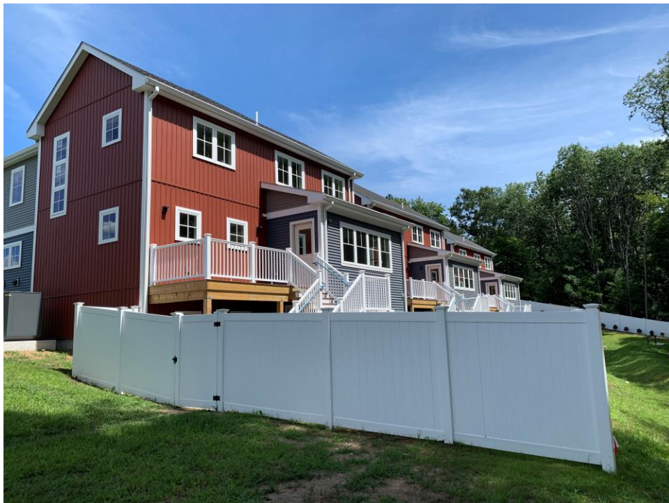
Typical rear of building and Privacy Fence (Bldg. C1)
