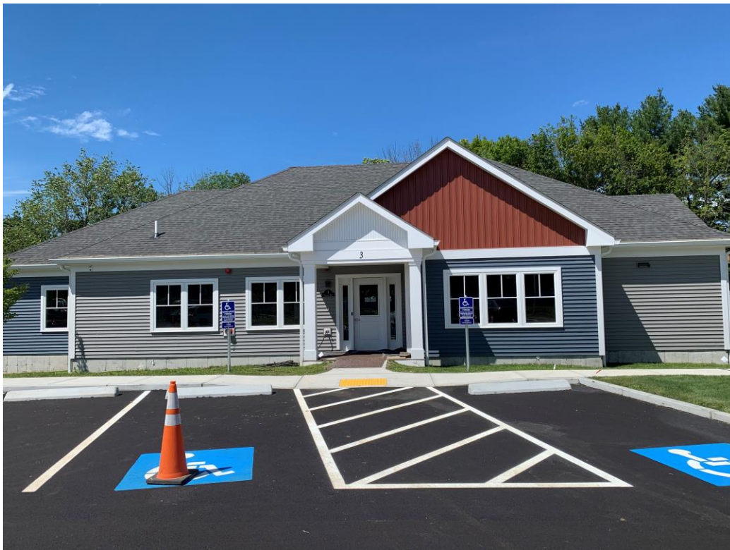
Building A-1 and typical accessible parking
