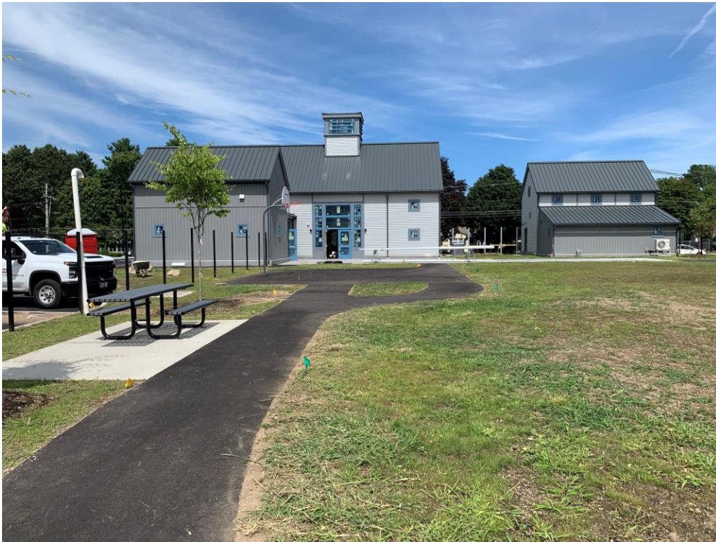
Typical Bit Walkway within the Common Area
