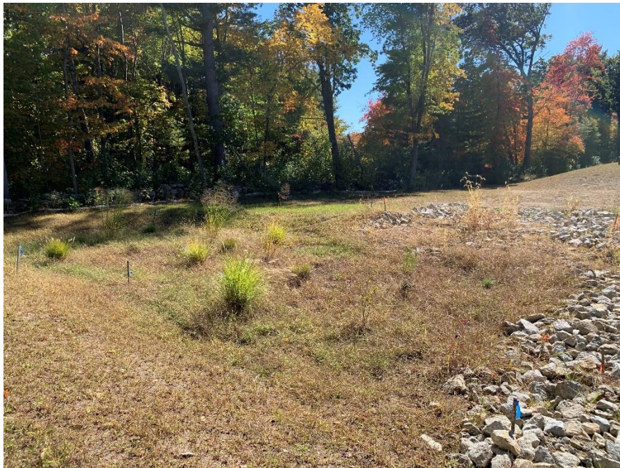
Completed rain garden area
