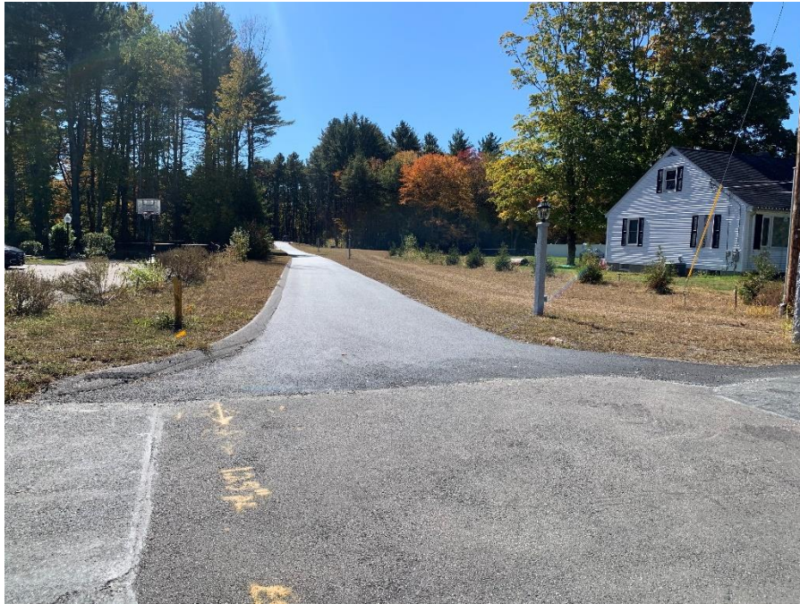
Subdivision roadway, showing top course and Cape Cod Berm
