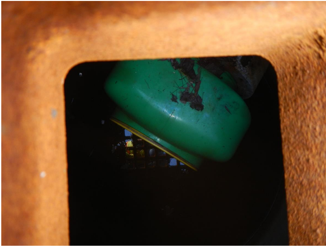
Installed CB hood
