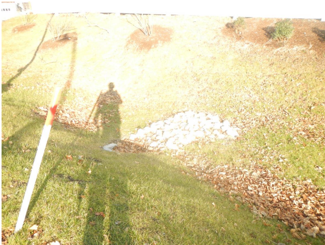
Typical rip rap installation
