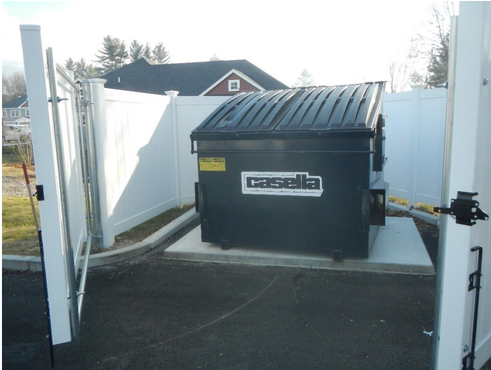
Concrete dumpster pad installed.
