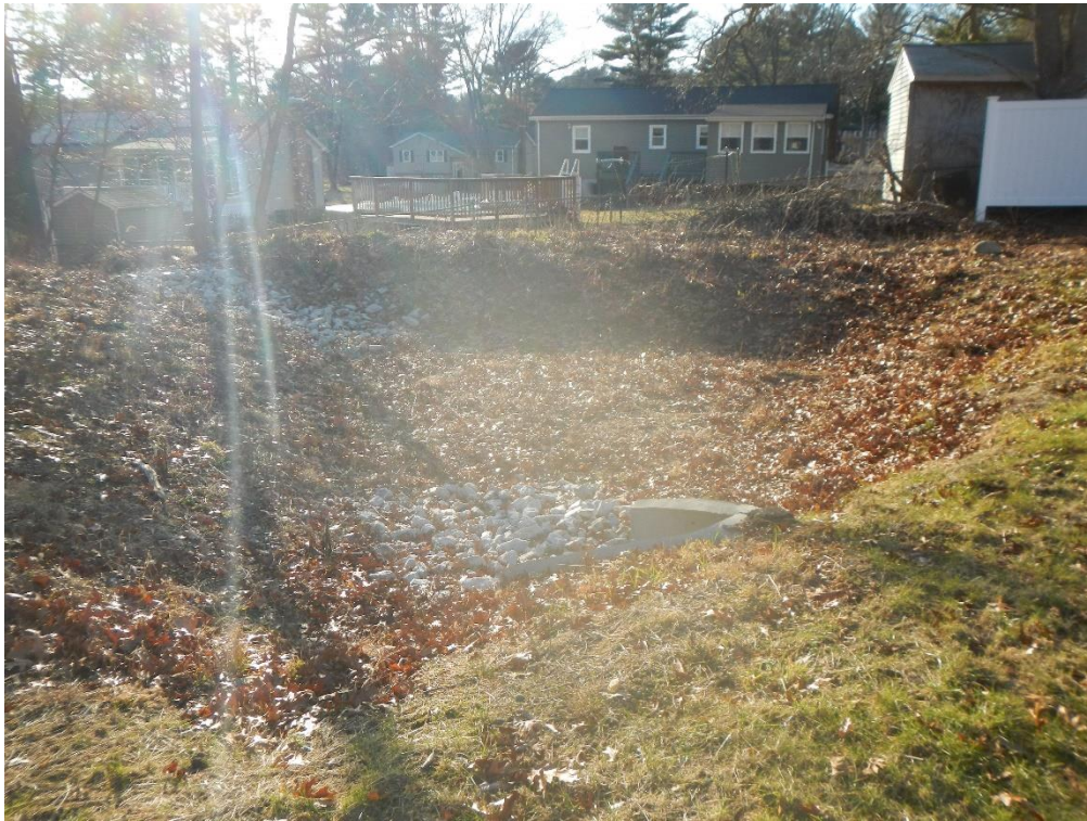
Infiltration basin that has been maintained
