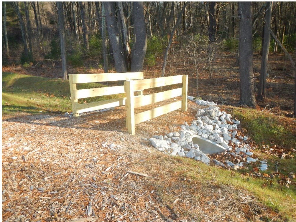
Railings added along footbridge
