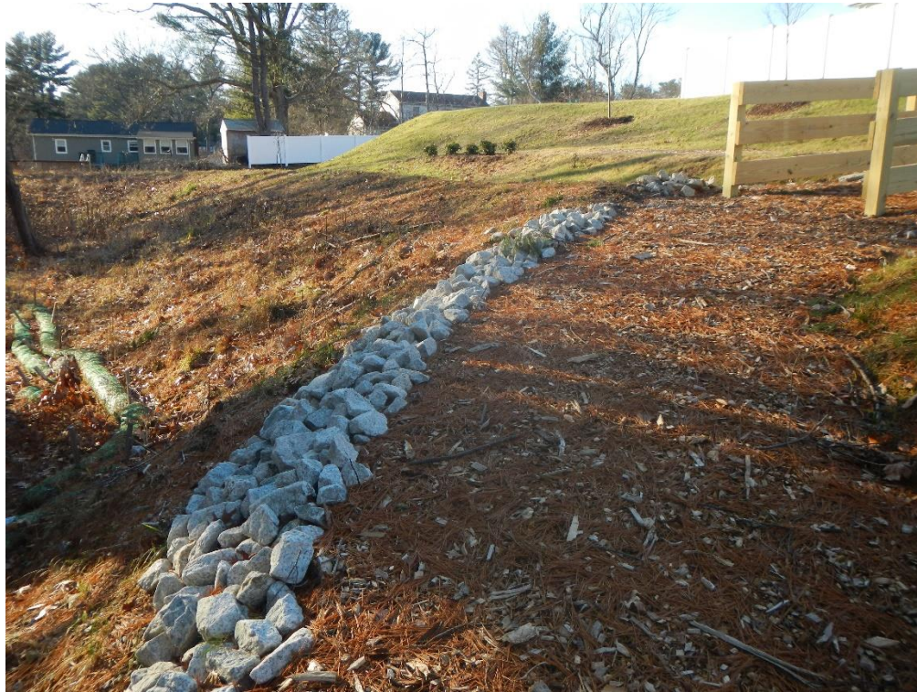
Stabilized slope along walking path
