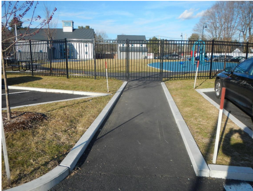
Fencing and playground equipment installed
