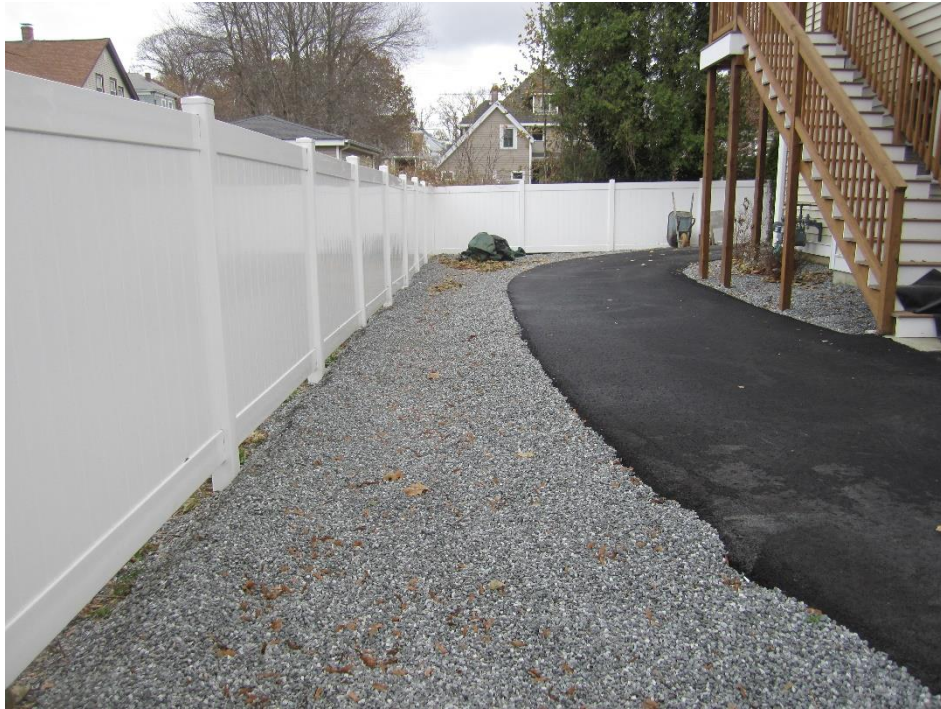
Typical swale area with stone installed in place of grass (photo 11/11/20)
