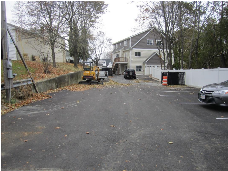
Typical parking area (photo 11/11/20)
