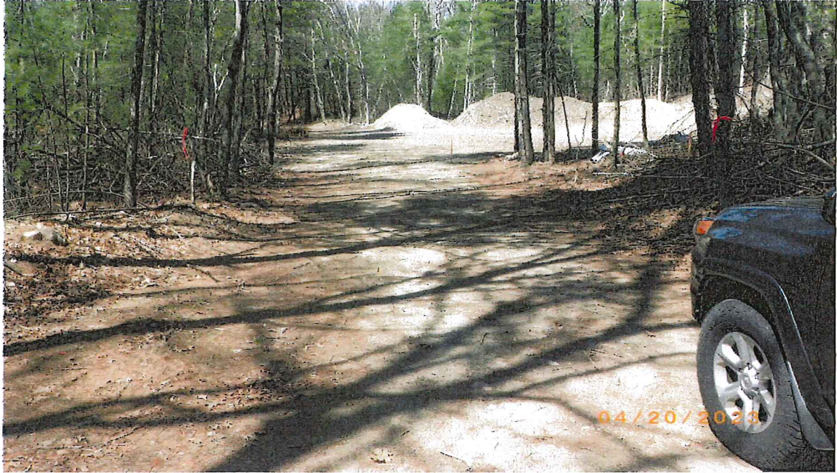
View to site interior along cleared access drive
