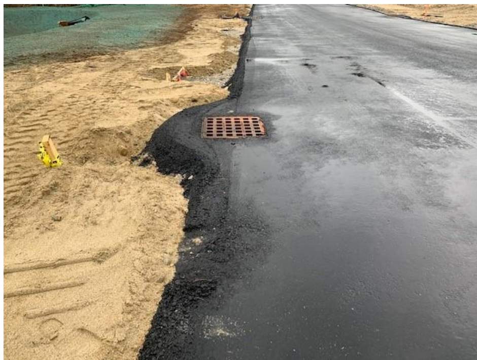
Typical Catch Basin with Dribble Berm
