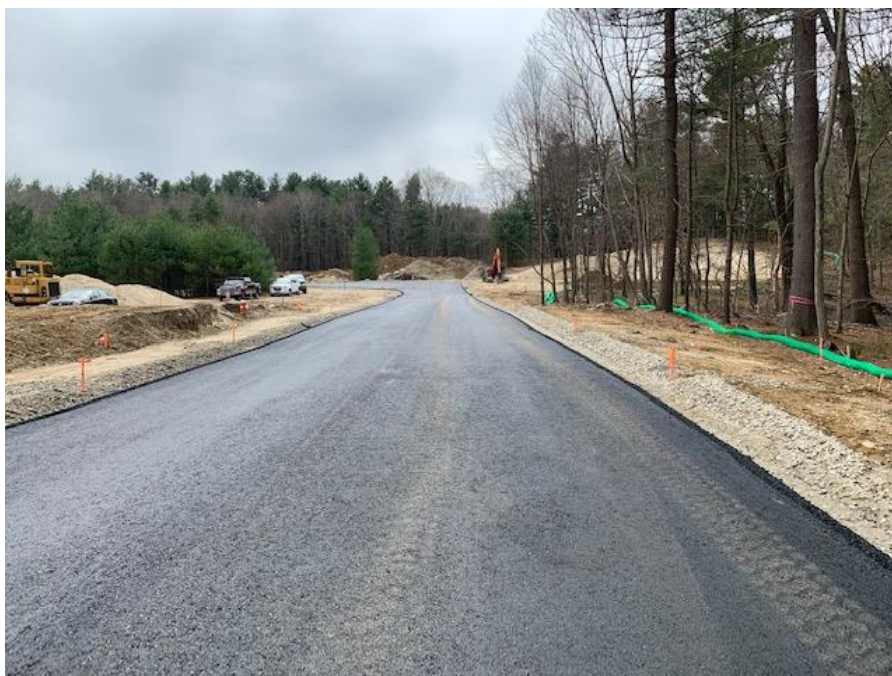
Typical Section of Paved Roadway with Dribble Berm
