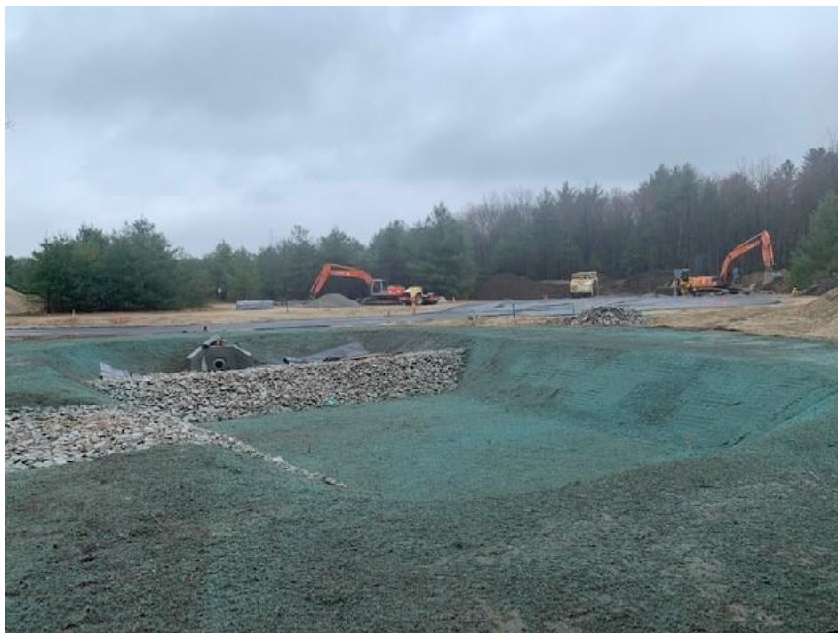
Infiltration Basin with Loam and Seed
