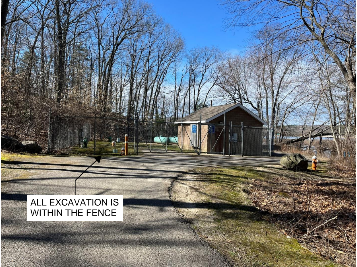
Photo 1: Wells Nos. 2, 2a, and 2b, view looking north.
