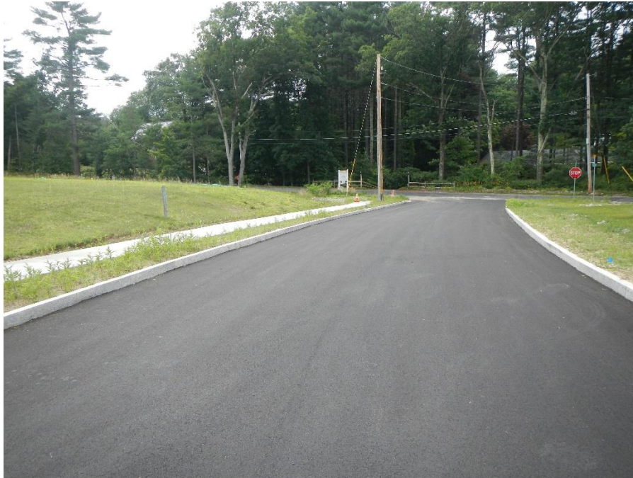
Typical roadway with top course completed
