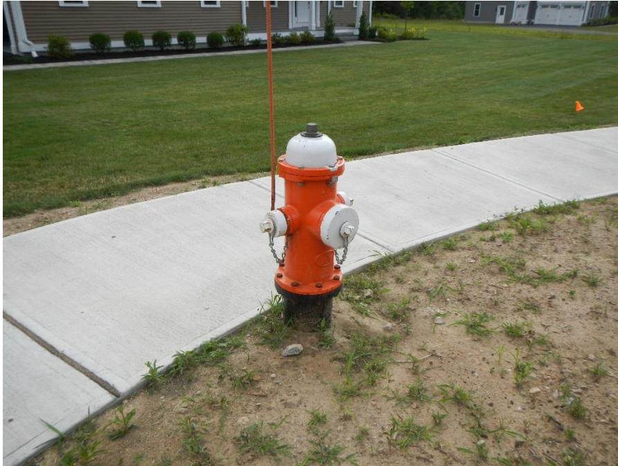
Hydrant that has been reset to proper grade and orientation
