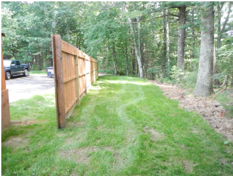
Installed screening fence
