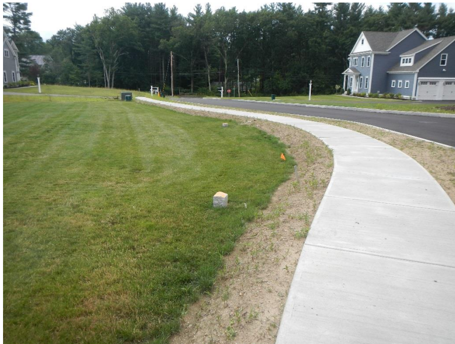
Sidewalk set approx. 12" above grade of adjacent lawn areas
