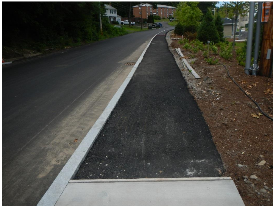
Guardrail has not been installed along Dean Avenue
