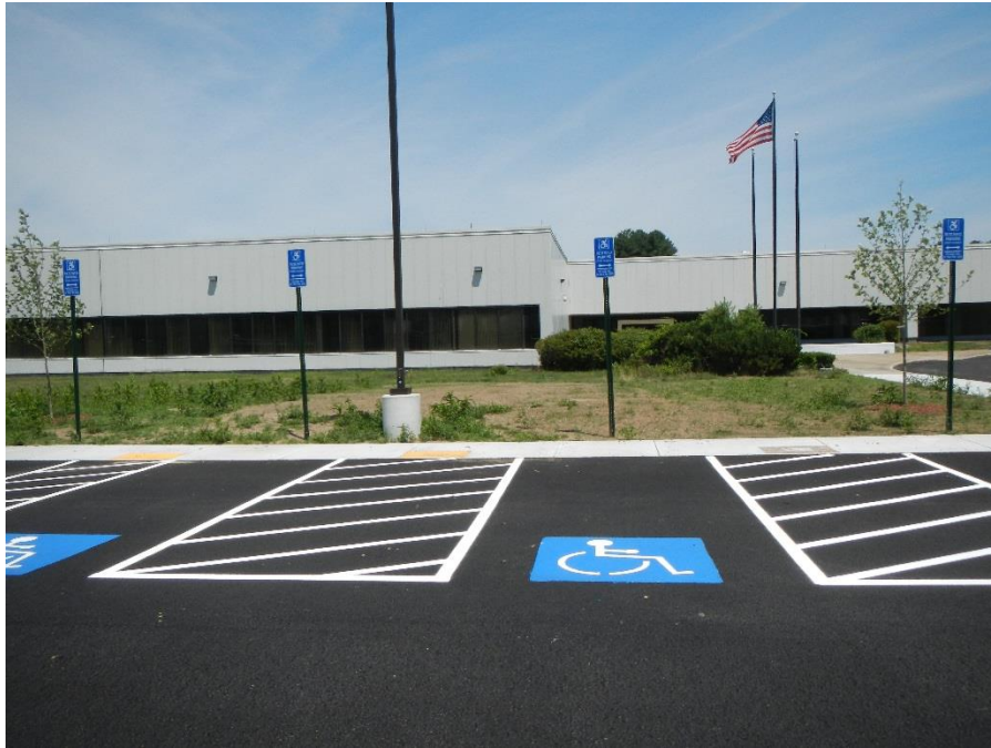
Typical accessible parking area
