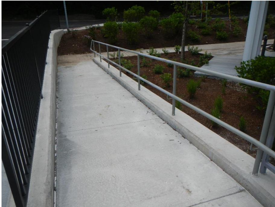
Installed accessible railings at Building 1
