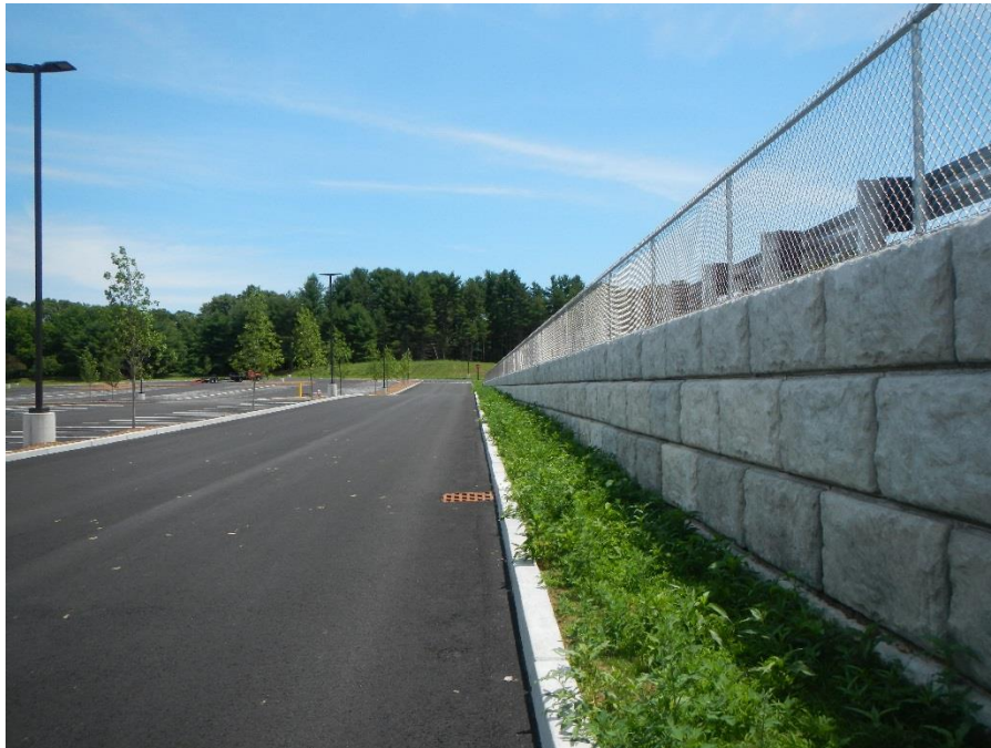
Retaining wall adjacent to site driveway
