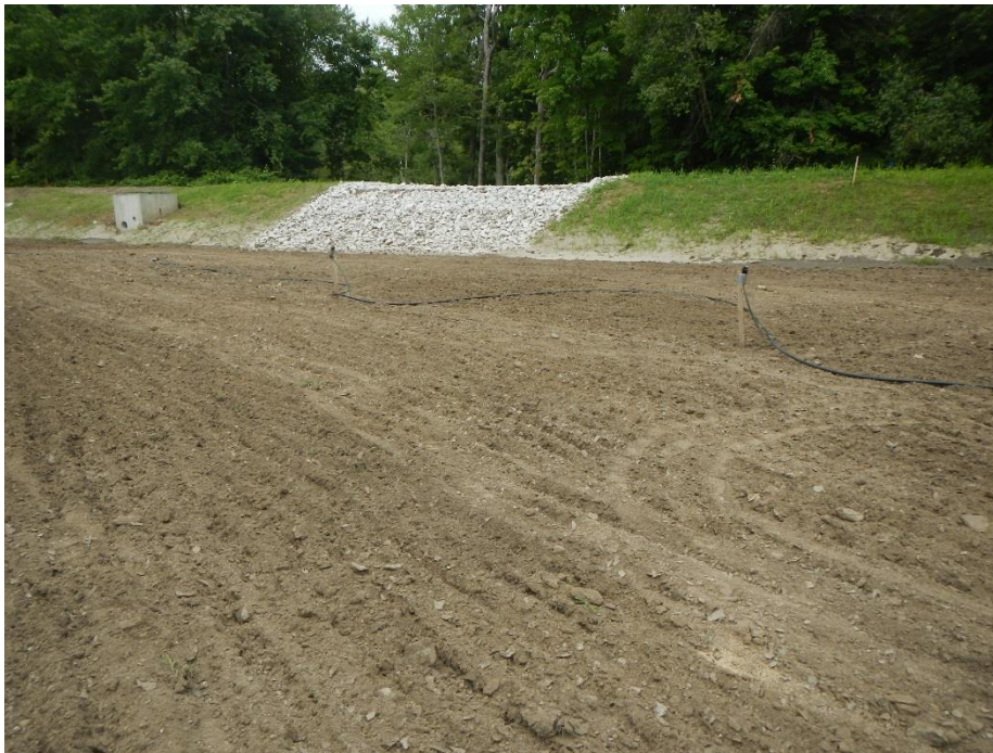
Infiltration basin with soils scarified and seeded
