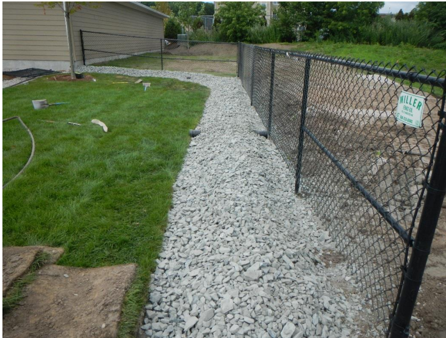
Gravel berm revised to crushed stone for stability.
