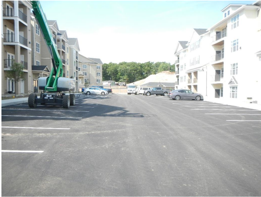
Typical paved parking area (Buildings 3 and 4)
