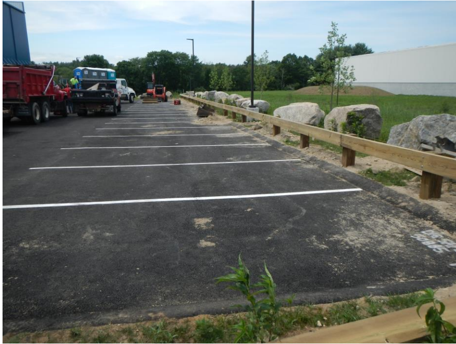
Partially installed timber guardrail
