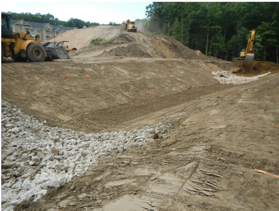
Sediment Forebay 2A under construction
