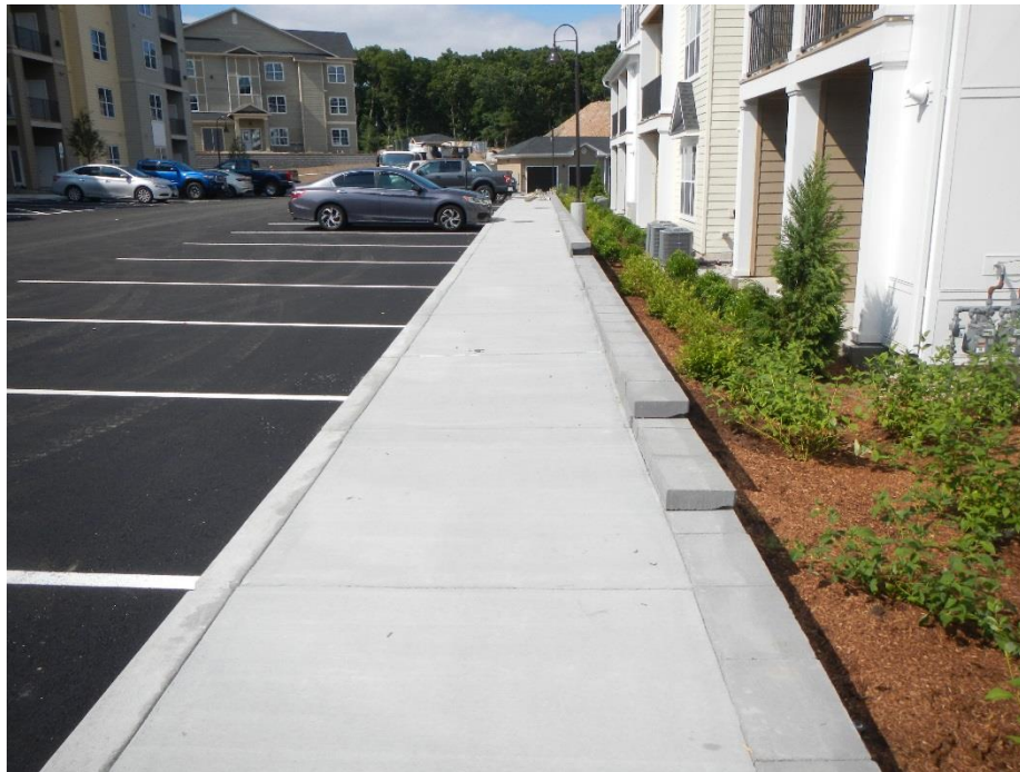
Retaining wall at Building 4 that requires fence installation
