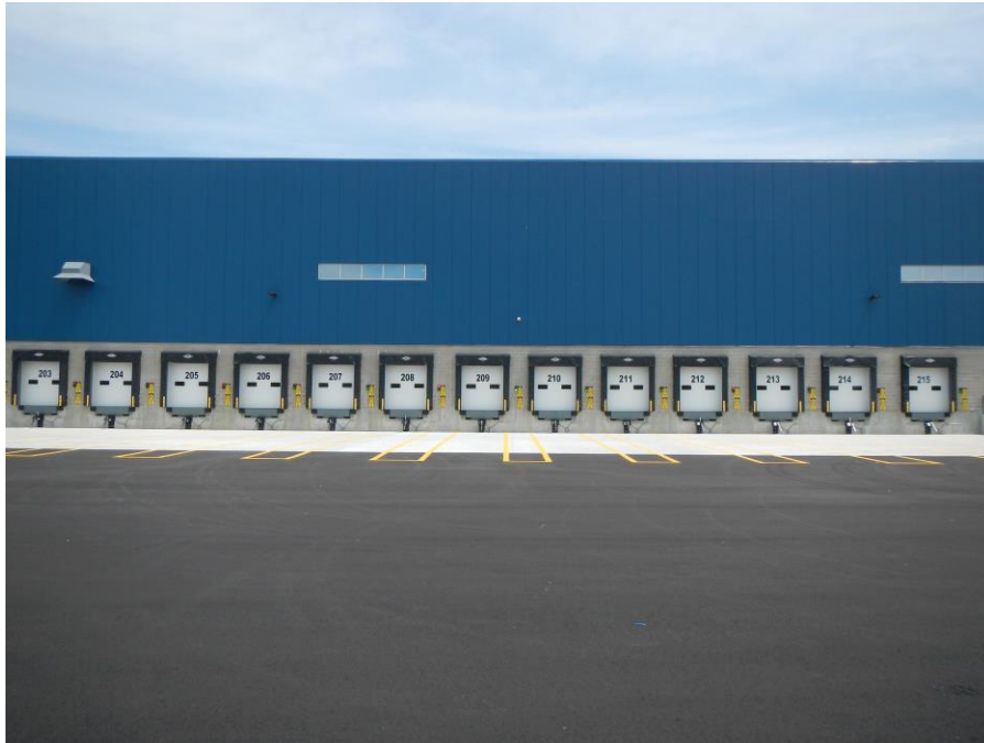
Typical loading dock area
