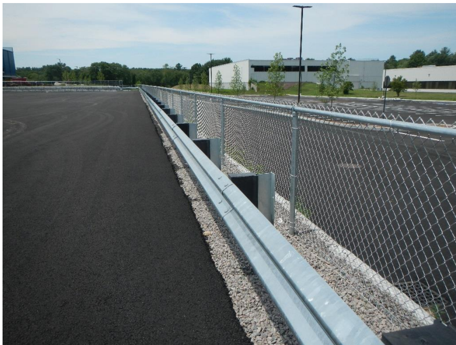
Guardrail and fall protection fence set on retaining wall
