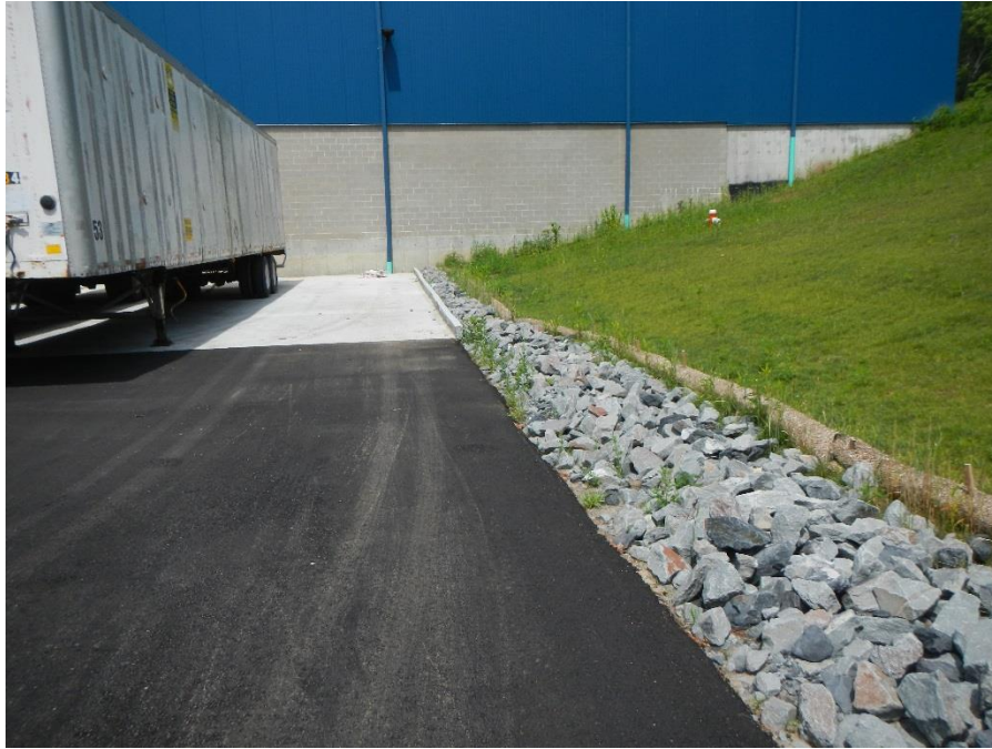
Rip rap installed at interface of loading area and adjacent slope
