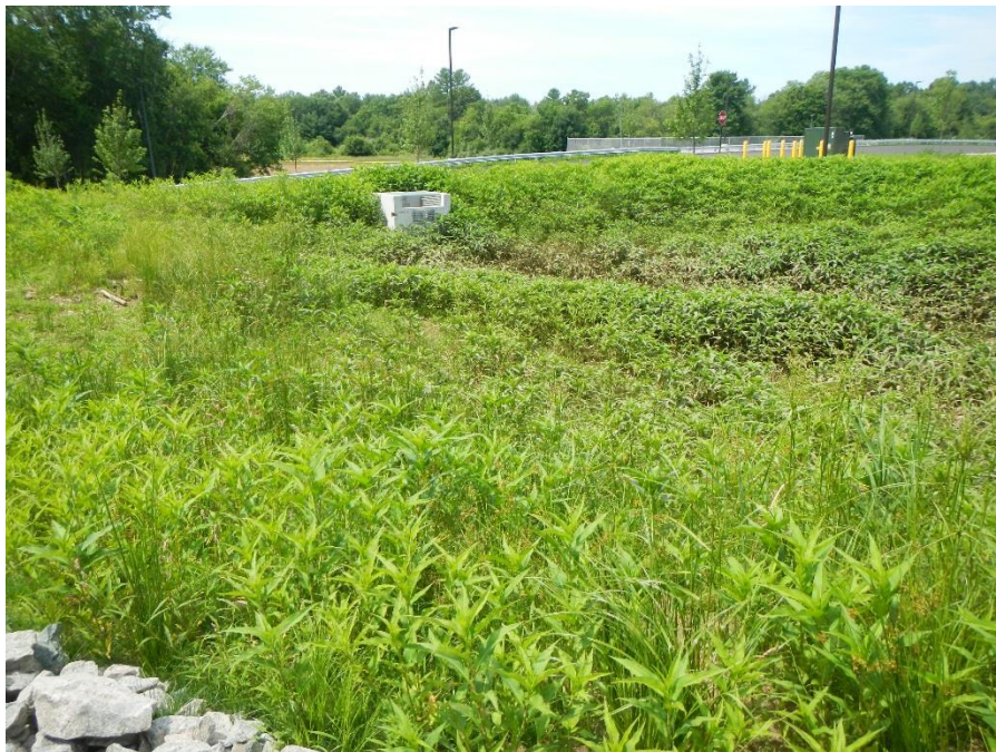
Infiltration basin dry after recent rainfall
