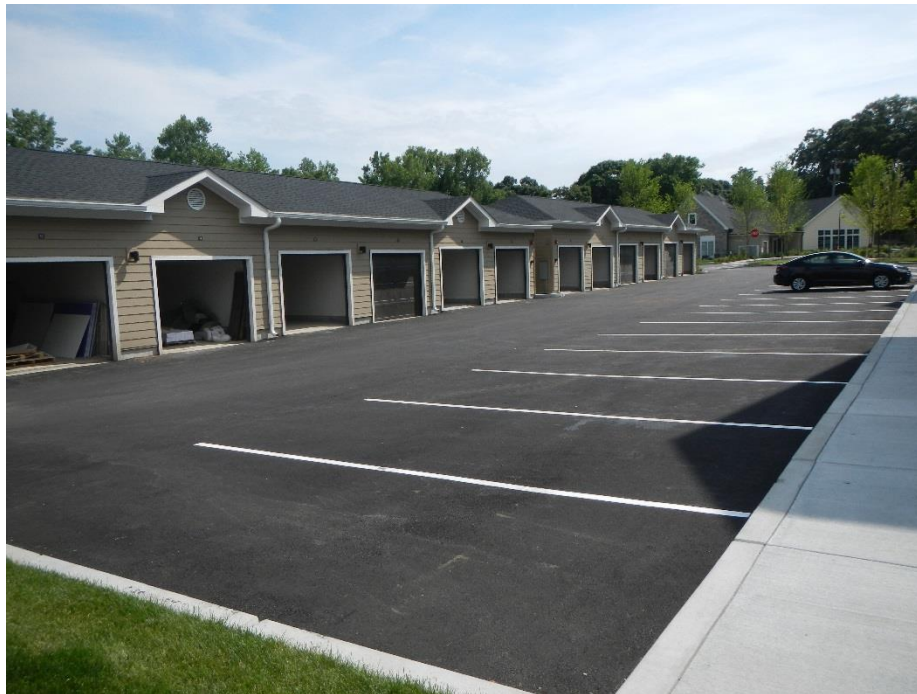
Typical paved parking area (Building 1)
