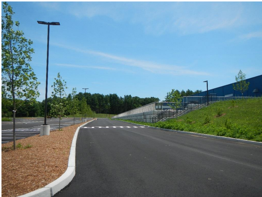
Site driveway with precast curb
