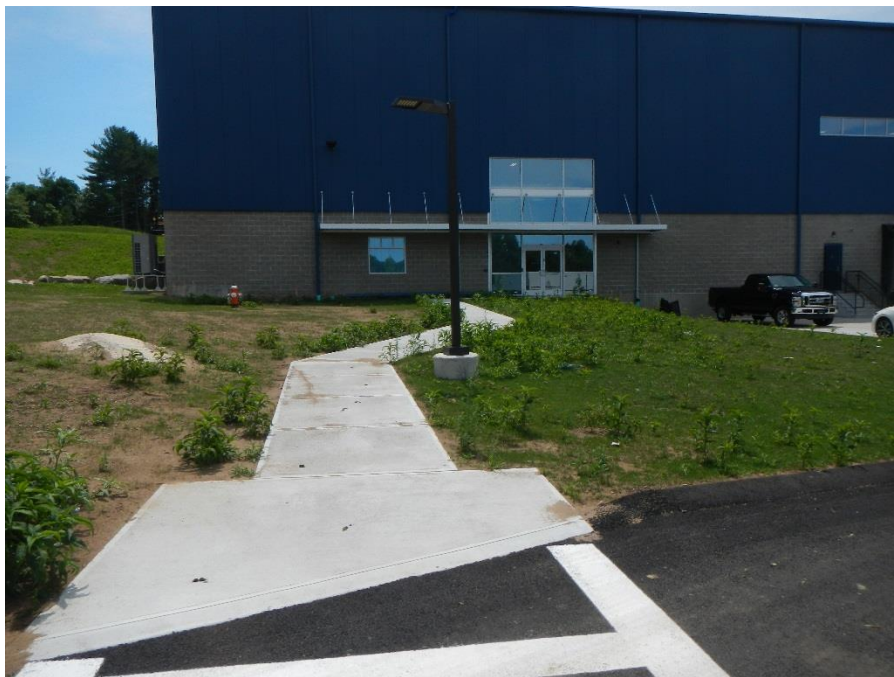
Concrete sidewalk connection to warehouse
