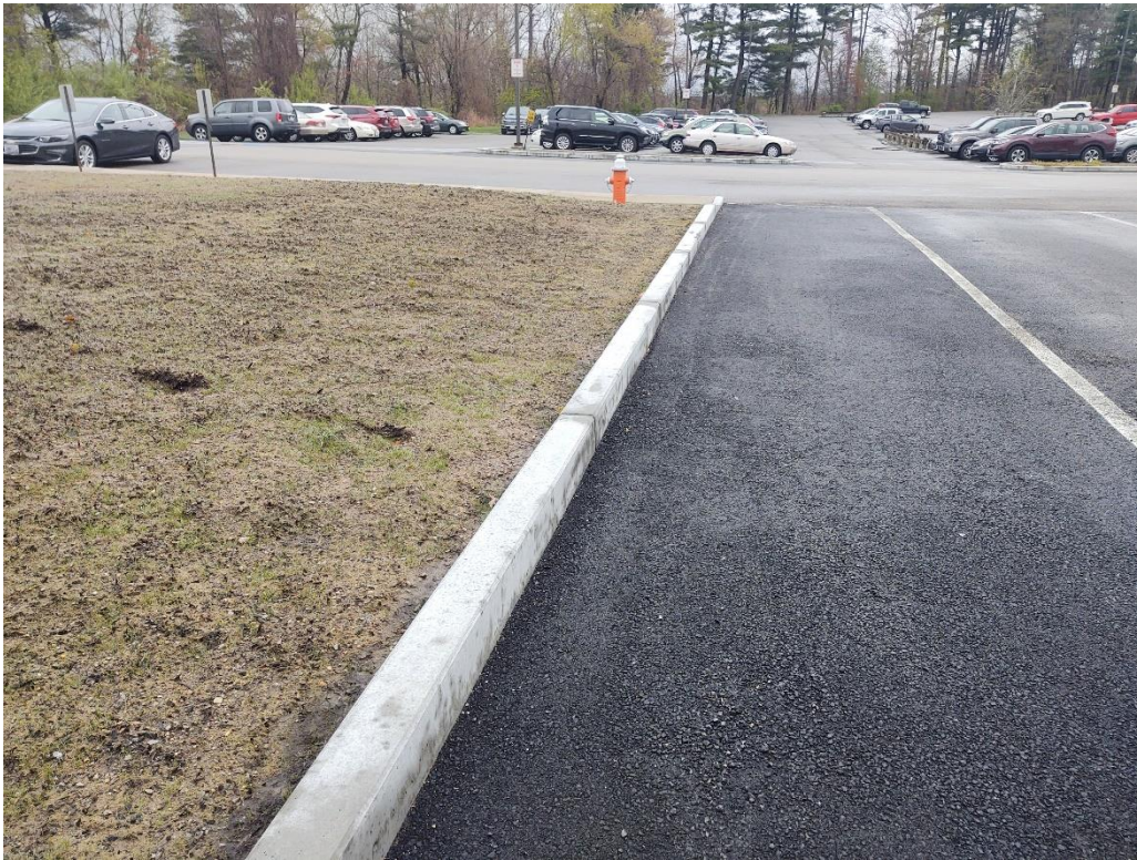
Typical precast reinforced concrete curb installation
