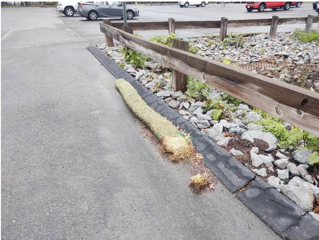
Erosion control remnants that require removal
