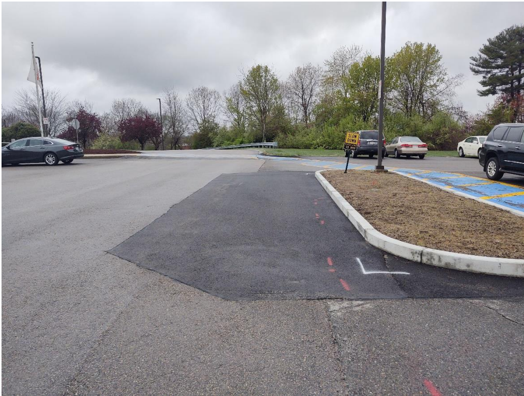
Typical pavement placement at former parking island
