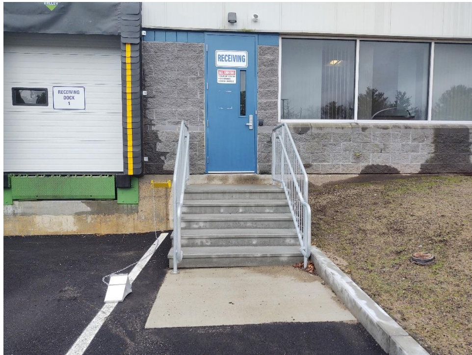
New stairs and access to building
