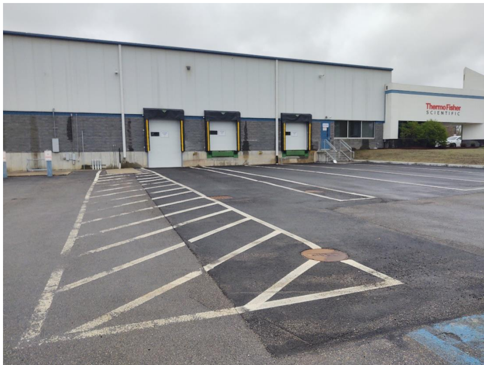
Modified loading dock area
