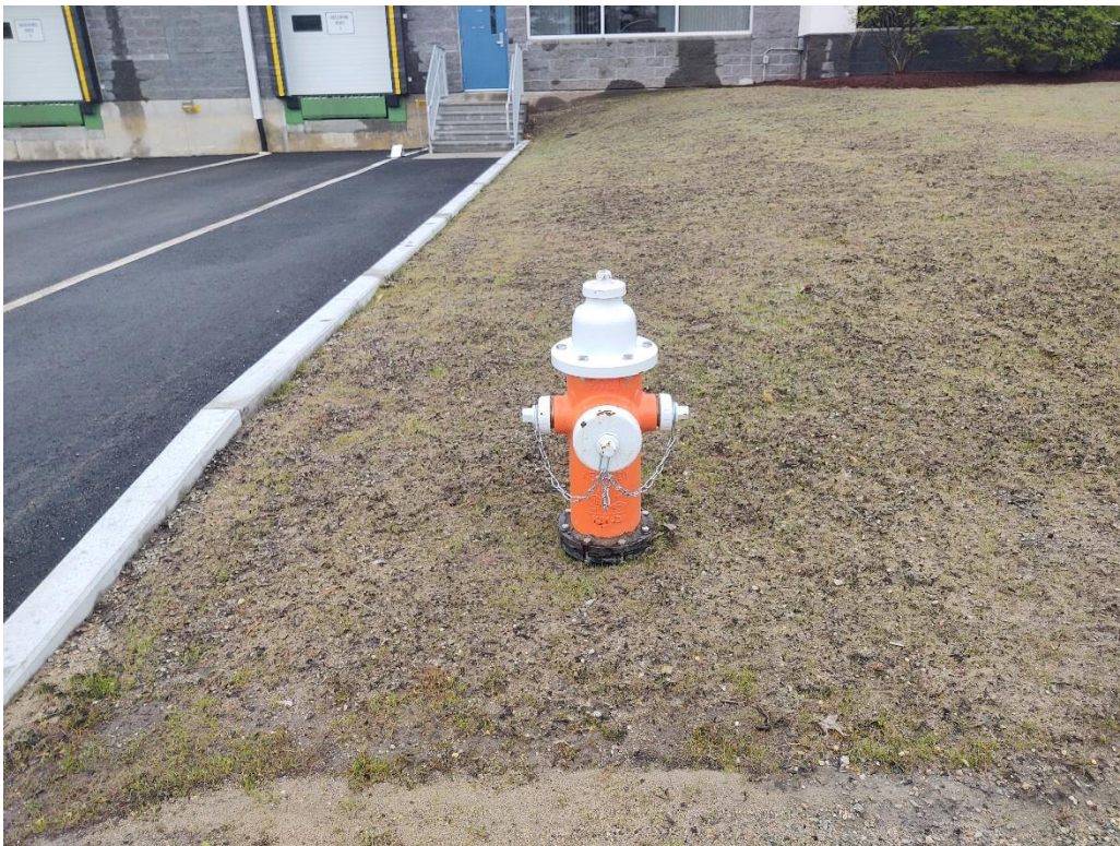
Factory painted fire hydrant and typical seeding in landscape area
