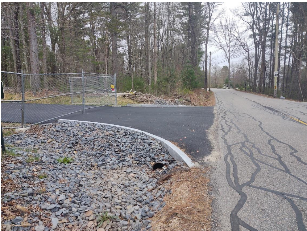
Typical granite curbing and ductile iron culvert at site entrance
