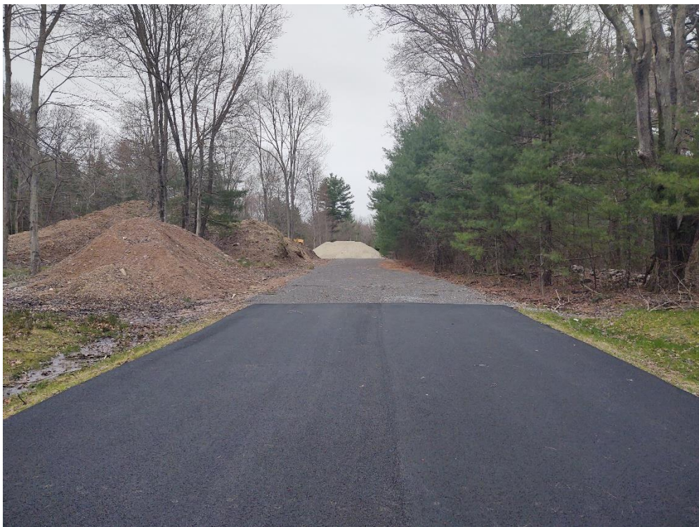
Gravel surface located beyond limits of paving
