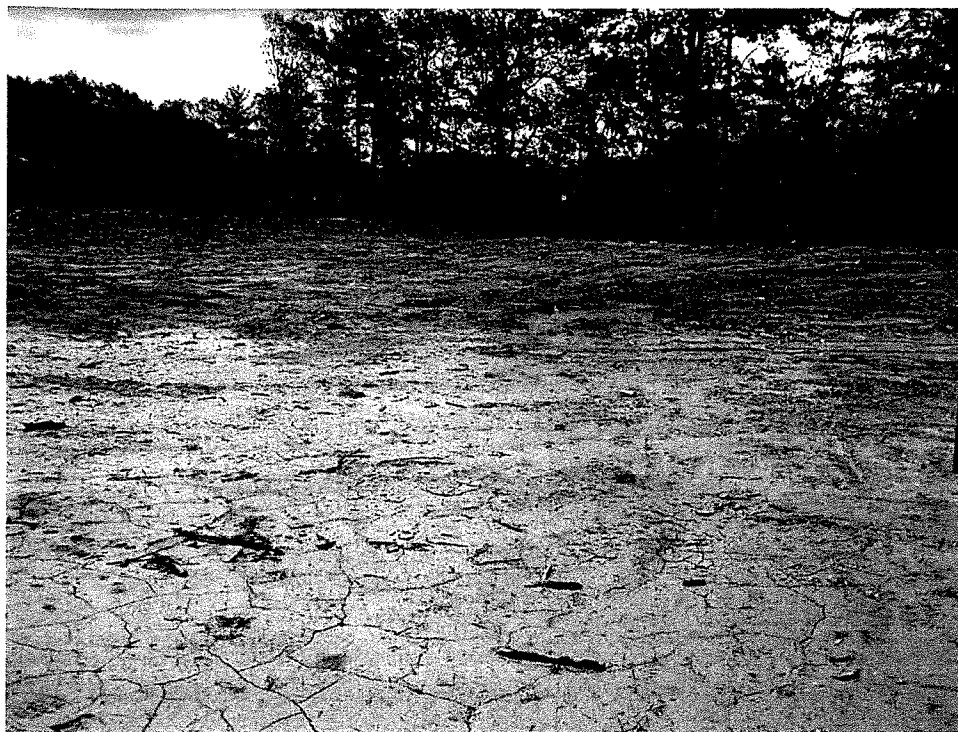
Lack of vegetation in stormwater detention area (southwest corner of site)
