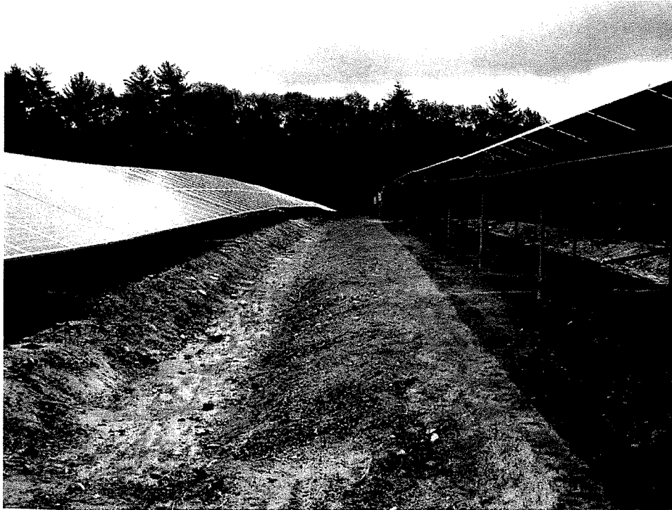
Typical vegetative cover at racking system swales
