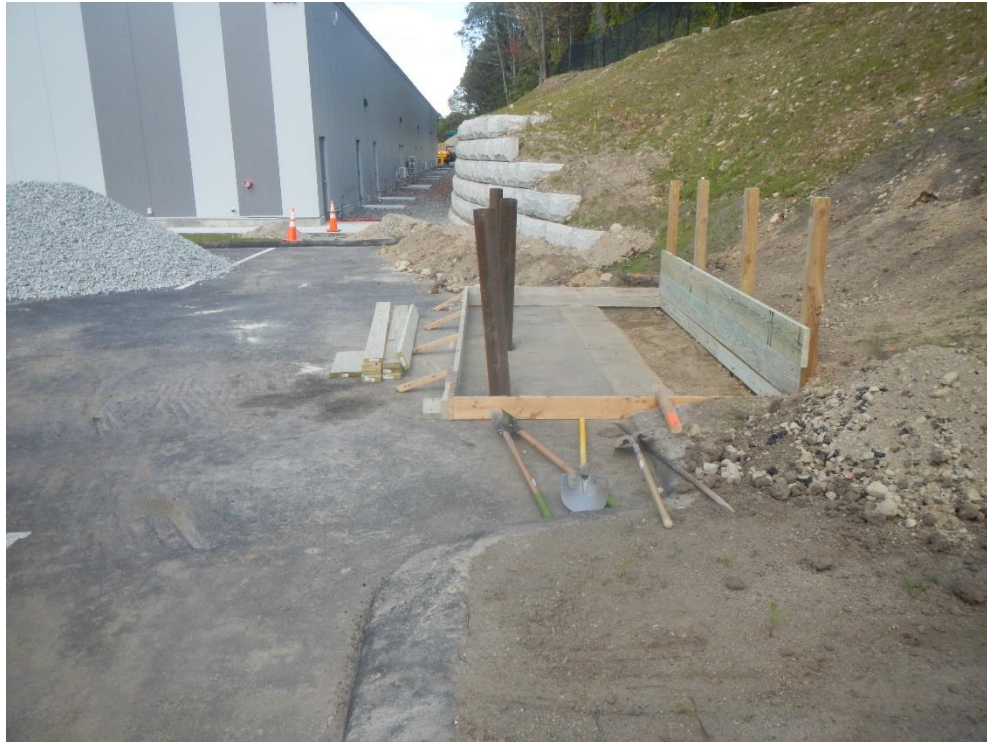
Propane tank storage area under construction
