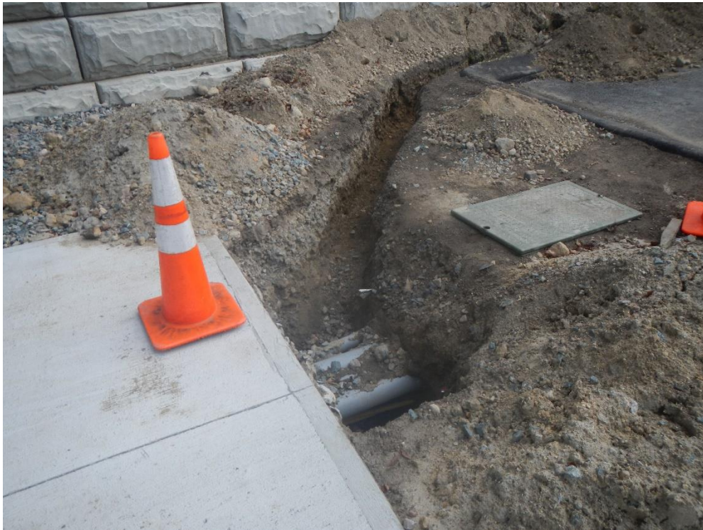
Trench adjacent to southerly walk
