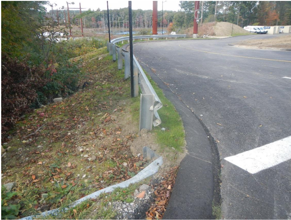
Guardrail installed at site entrance
