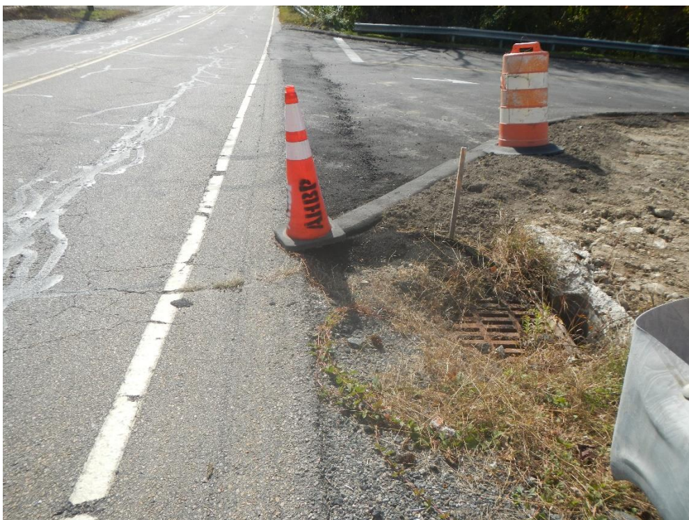
Catch basin located behind existing bituminous berm
