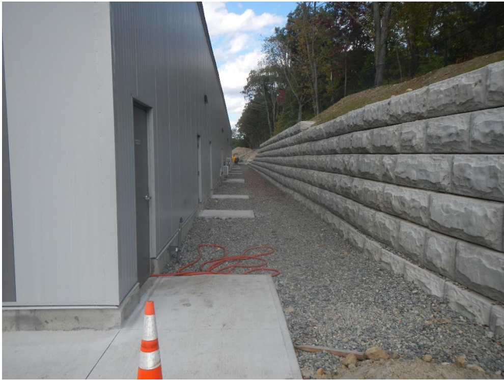
Block retaining wall with chain link fence at top of slope
