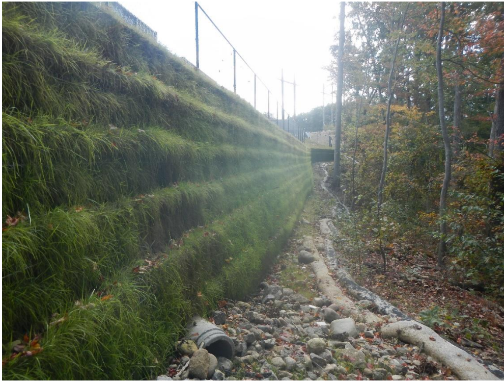
Westerly retaining wall
