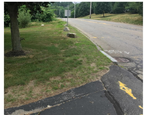
Figure 1: Looking to the south from site driveway
