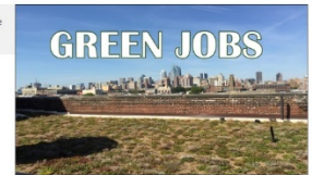
This green roof in Philadelphia, Pennsylvania is an example of a green job opportunity in your community.
