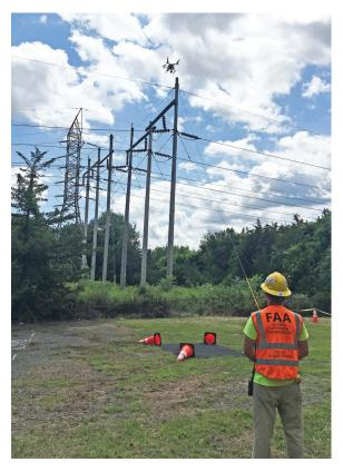
Drones are flown by a two-person crew in rights of way — one person operates the drone (shown here) and the other keeps the drone operator informed of any special conditions or hazards during the inspections.
