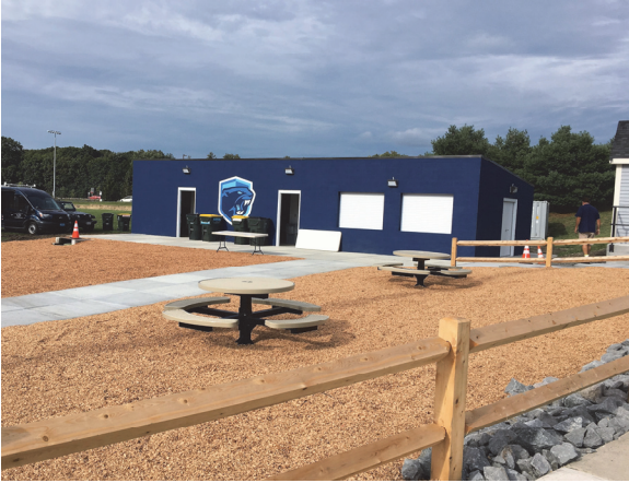
New concession and restroom facility at FHS
