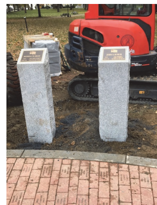
Pedestals are installed.
