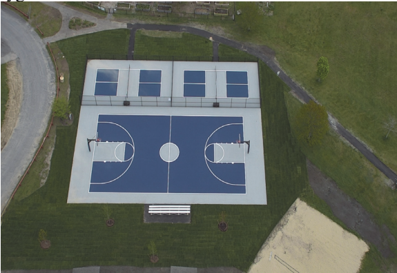
New pickleball and basketball courts at King Street Memorial Park.
