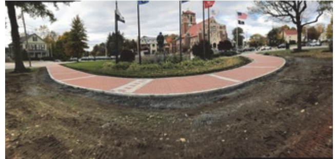
Brick work is completed
