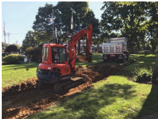
Beginning the walkway project
