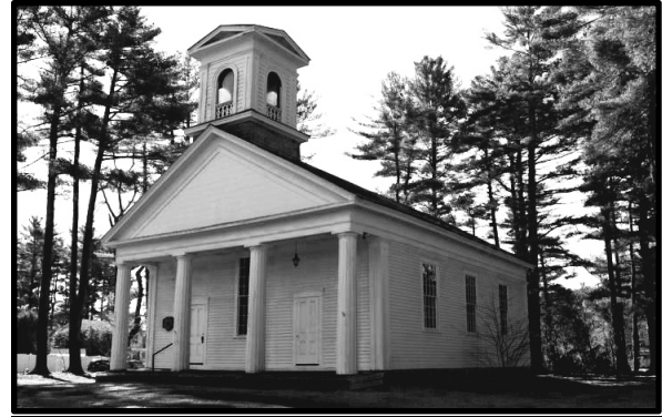
(South Franklin Congregational Meeting House)
