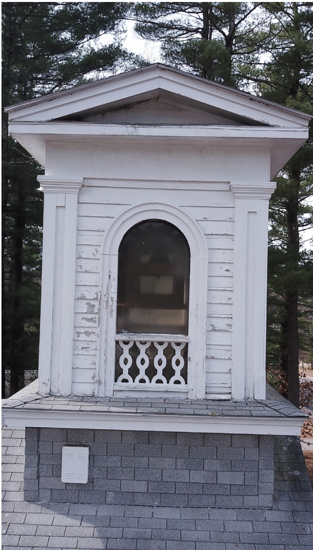
Paint loss at cupola exposing wood siding and trim. A number of siding pieces have split horizontally.
