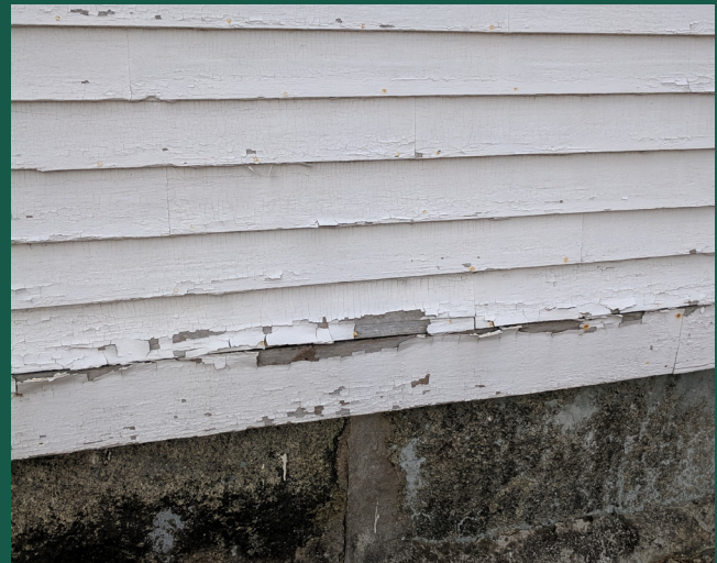
Paint loss at the bottom most siding and trim board.
