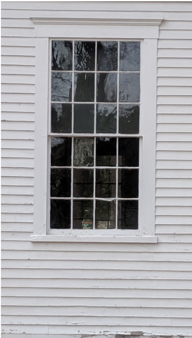
Exterior picture of typical 12 over 12 window. Notice the damaged muntin rail referenced on opposite page.
