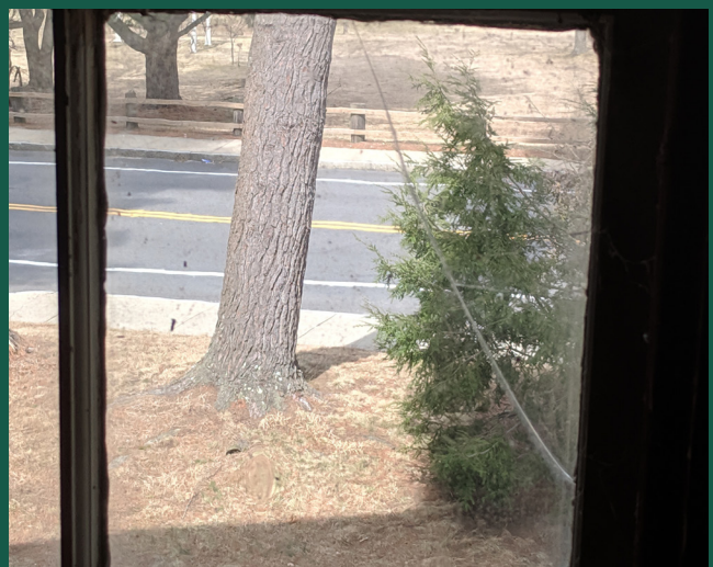
Evidence of cracked light at second floor window.
