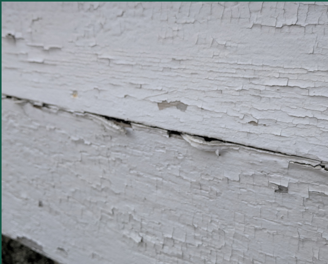
Detail photo at siding lap joint, observed flaking, craquelure paint.
