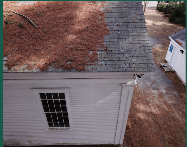
Significant pine needle and tree branches have fallen and are collecting on the west rear roof.
