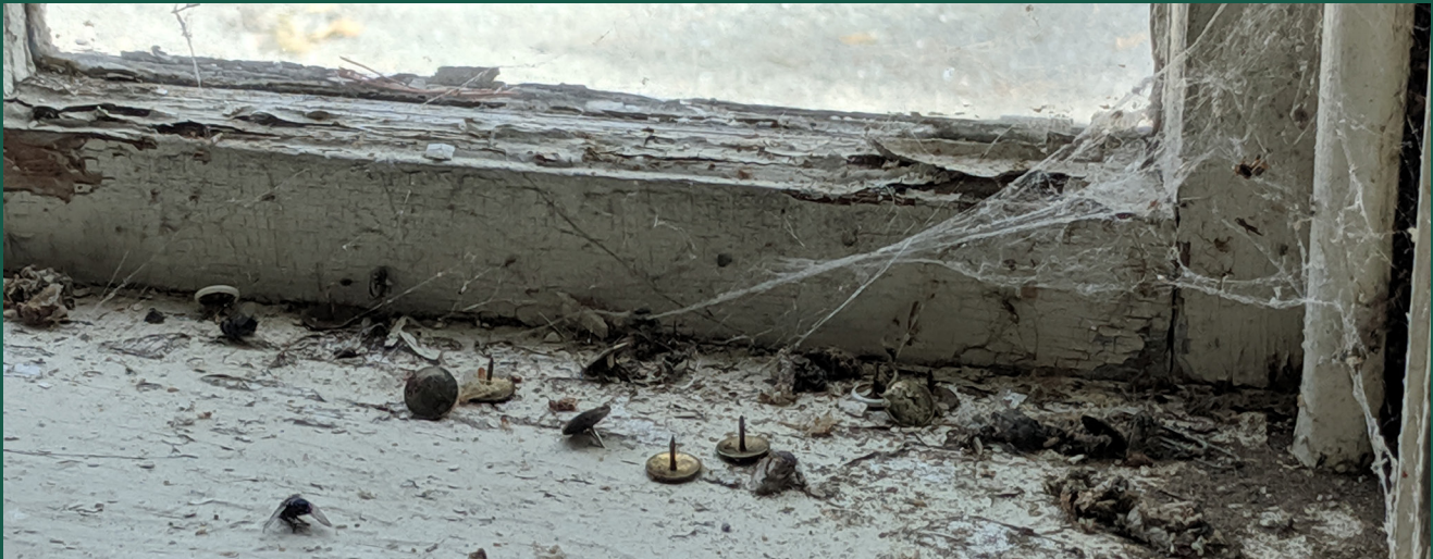
Evidence of water damage and paint loss at window sill on east side.
