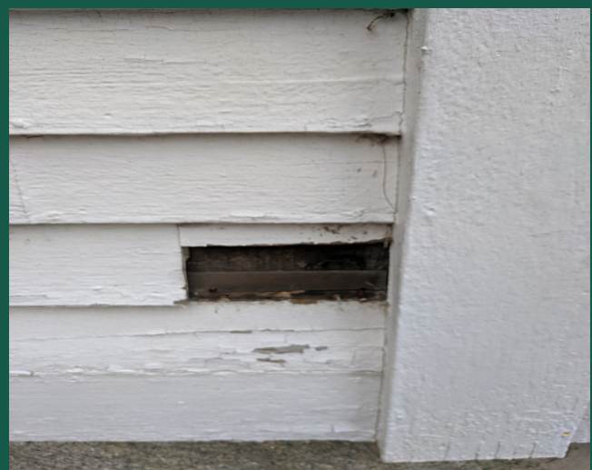
Missing siding piece exposing sheathing behind.
