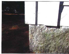
Photo C.2 – Corner Board and Granite Foundation
