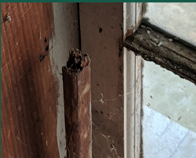
The sash stile show signs of wear and damage at second floor. Sash bars are also deteriorating.
