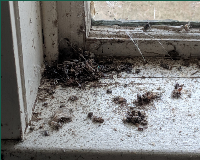
Close up detail at a window sill (typical) showing pest and animal waste.
