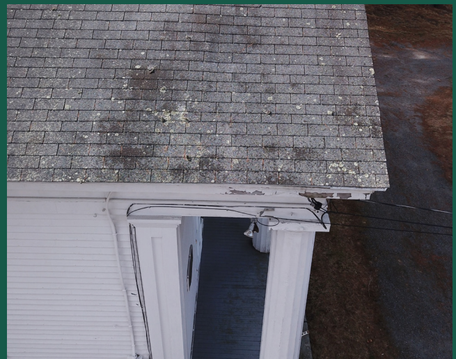
Algae, moss and lichens visible on the main roof, east side front.
