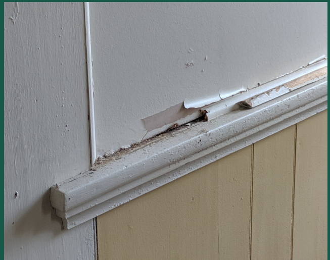
Cracked and peeling paint at wood trim in main assembly room.
