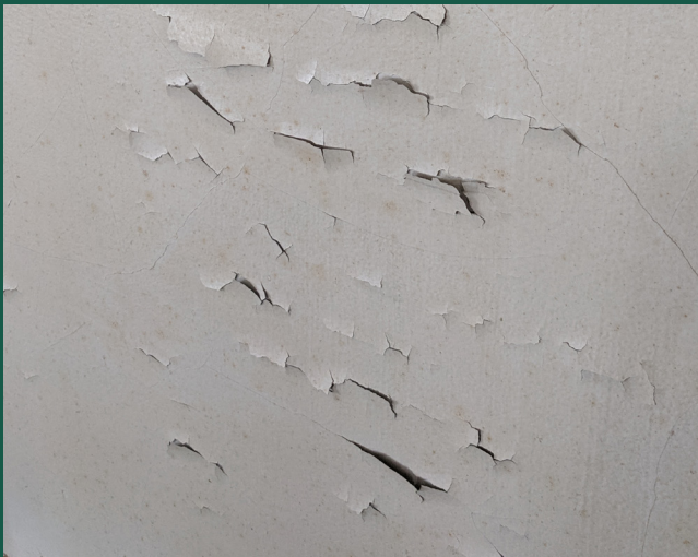
Paint cracking and peeling in main assembly room.
