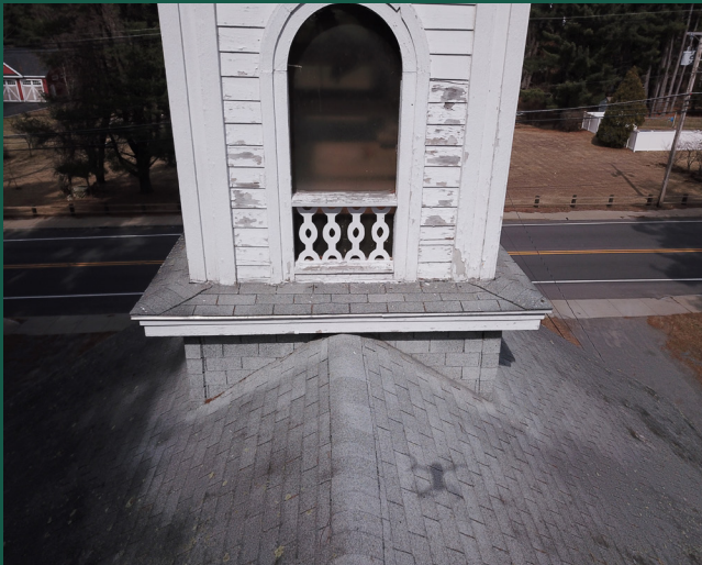
Close up detail at the cupola and main roof connection. Note slight granular loss occurring on most shingles due to age.
