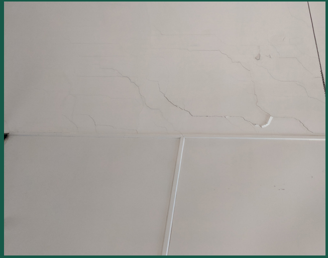
Close up detail at the ceiling showing paint and plaster cracks.
