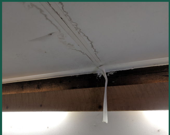
Apparent water damage to ceiling panel at second floor.
