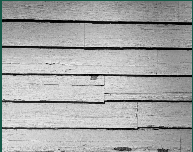
A number of horizontal splits occurring in the siding can be observed as well as paint loss.
