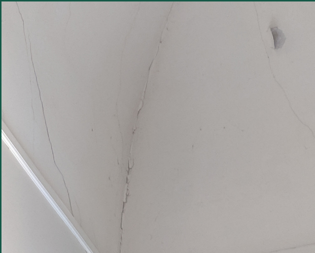
Close up detail at the ceiling showing paint and plaster cracks.
