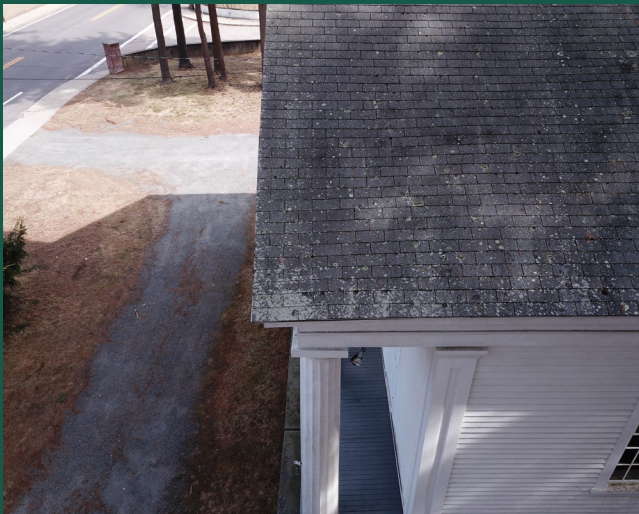
Algae, moss and lichens visible on the main roof, west side front.
