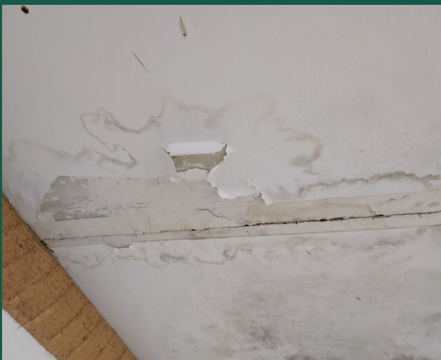
Apparent water damage and peeling paint at second floor.
