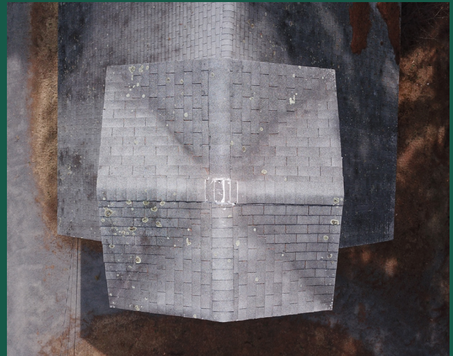
Algae, moss and lichens visible on the cupola roof.
