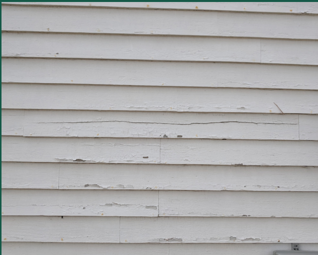
Horizontal split occurring in a siding board can be observed as well as paint loss.
