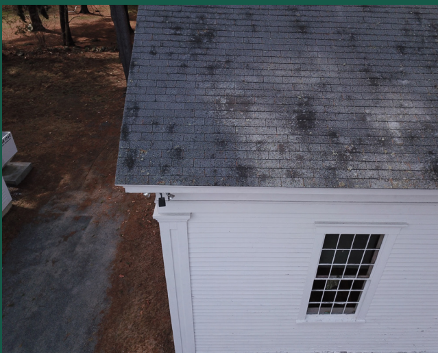
Algae, moss and lichens visible on the main roof, east side rear.
