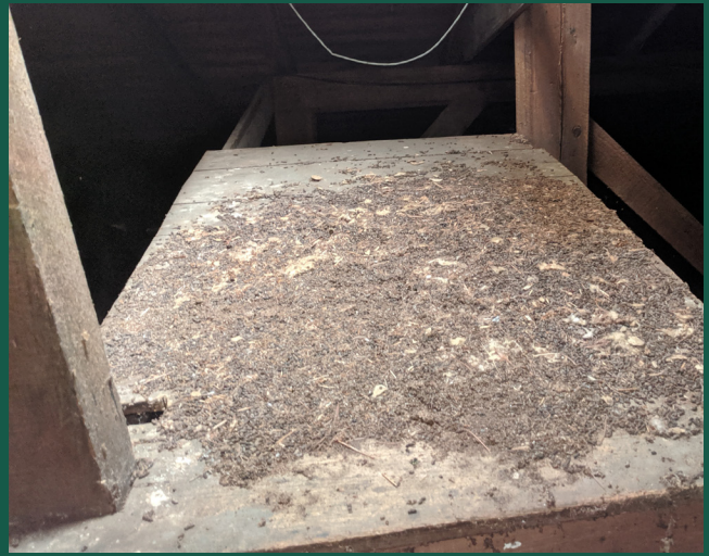
Observed bird droppings inside of the bell tower.
