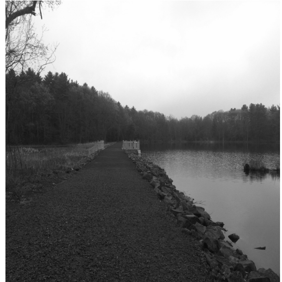
Dam Restoration, DelCarte Recreation Area
