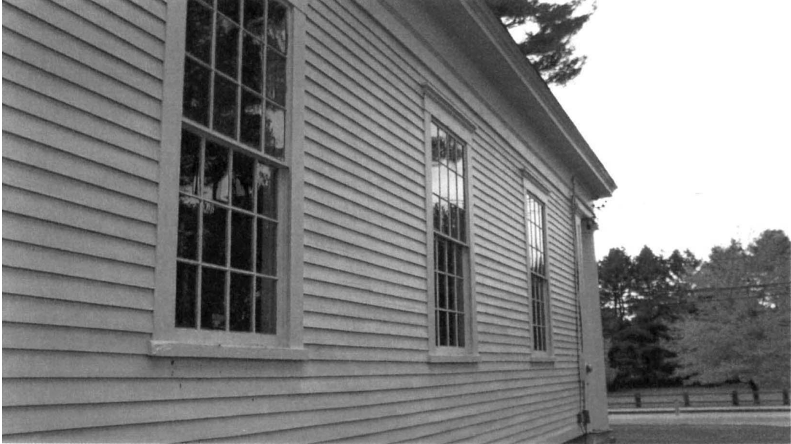
PHOTO 5. East Elevation – Window Details (2011).
