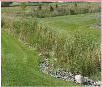
**Infiltration Trenches** - shallow excavations filled with stone. They can be designed to capture sheet flow or piped inflow. The stone provides underground storage for stormwater runoff. The stored runoff gradually exfiltrates through the bottom and/or sides of the trench into the subsoil and eventually into the water table.
