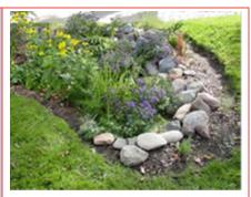
**Vegetated Swales** - vegetated open channels that are designed to provide for non-erosive stormwater conveyance that accents natural landscape.
