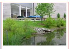
**Infiltration Basins** - Infiltration basins are stormwater runoff impoundments that are constructed over permeable soils. Pretreatment is critical for effective performance of infiltration basins. Runoff from the design storm, a critical rainfall event over a specified time period, is stored until it exfiltrates through the soil at the bottom of the basin.
