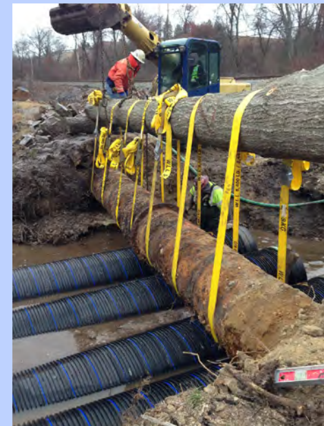
Emergency culvert replacement - 2014
