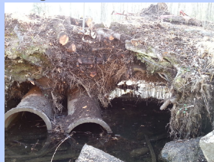
Culvert under the Beaver St interceptor (24" sewerline) on the verge of collapse - 2014
