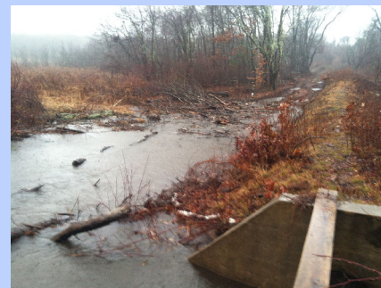
The failing culvert led to local flooding and risked dumping thousands of gallons of wastewater into a local waterway - 2014
