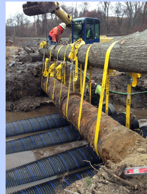
Emergency culvert replacement - 2014
